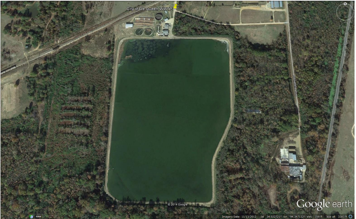
Figure 1. Google Earth image dated Nov 13, 2012 of overview of City of DeQueen's WWTP.
