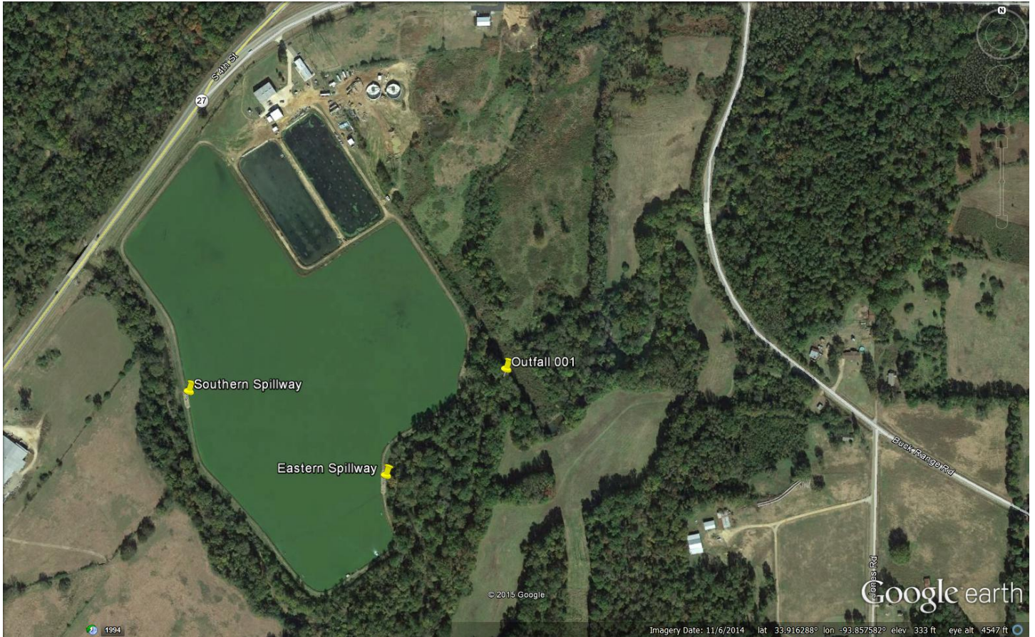
Figure 1. Google Earth image dated Nov 6, 2014 of Nashville WWTP, permitted outfall, and two spillways.
