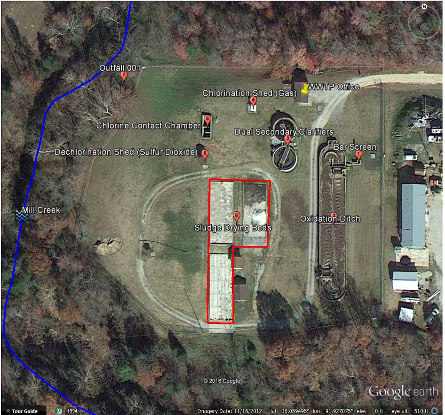
Figure 1. Aerial view of City of Melbourne WWTP and components (Google Earth: imagery date November 16, 2012).
