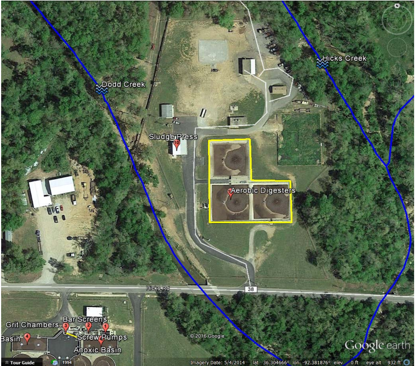
Figure 2. Aerial view of aerobic digesters and sludge press facility located just northeast of WWTP (Google Earth: imagery date May 4, 2014).
