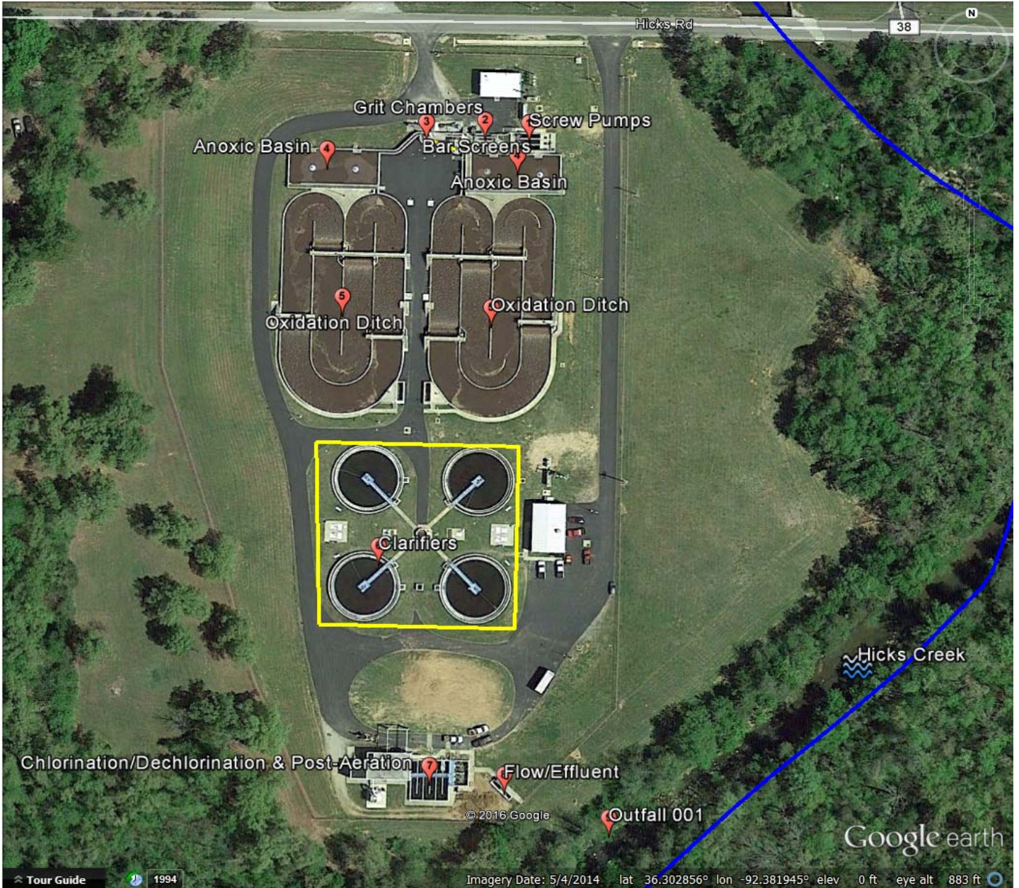
Figure 1. Aerial view of City of Mountain Home WWTP and associated components (Google Earth: imagery date May 4, 2014).
