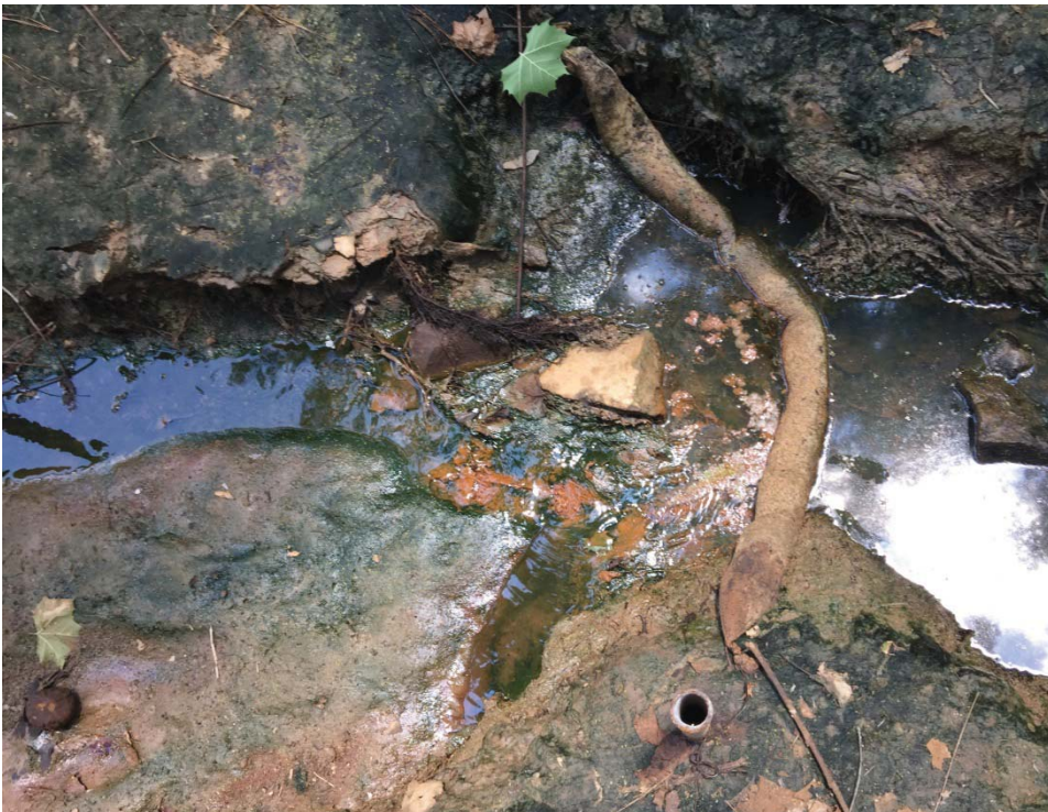
Sock initially installed day of inspection after removing oil sheen
