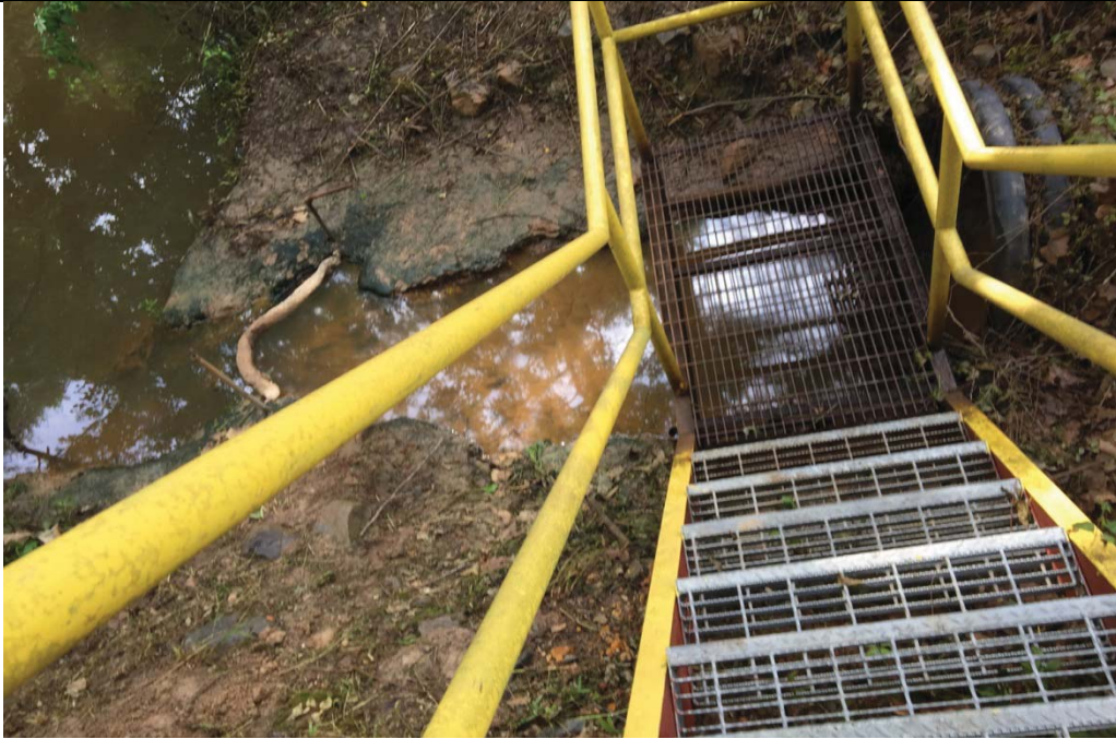
Sock initially installed day of inspection after removing oil sheen
