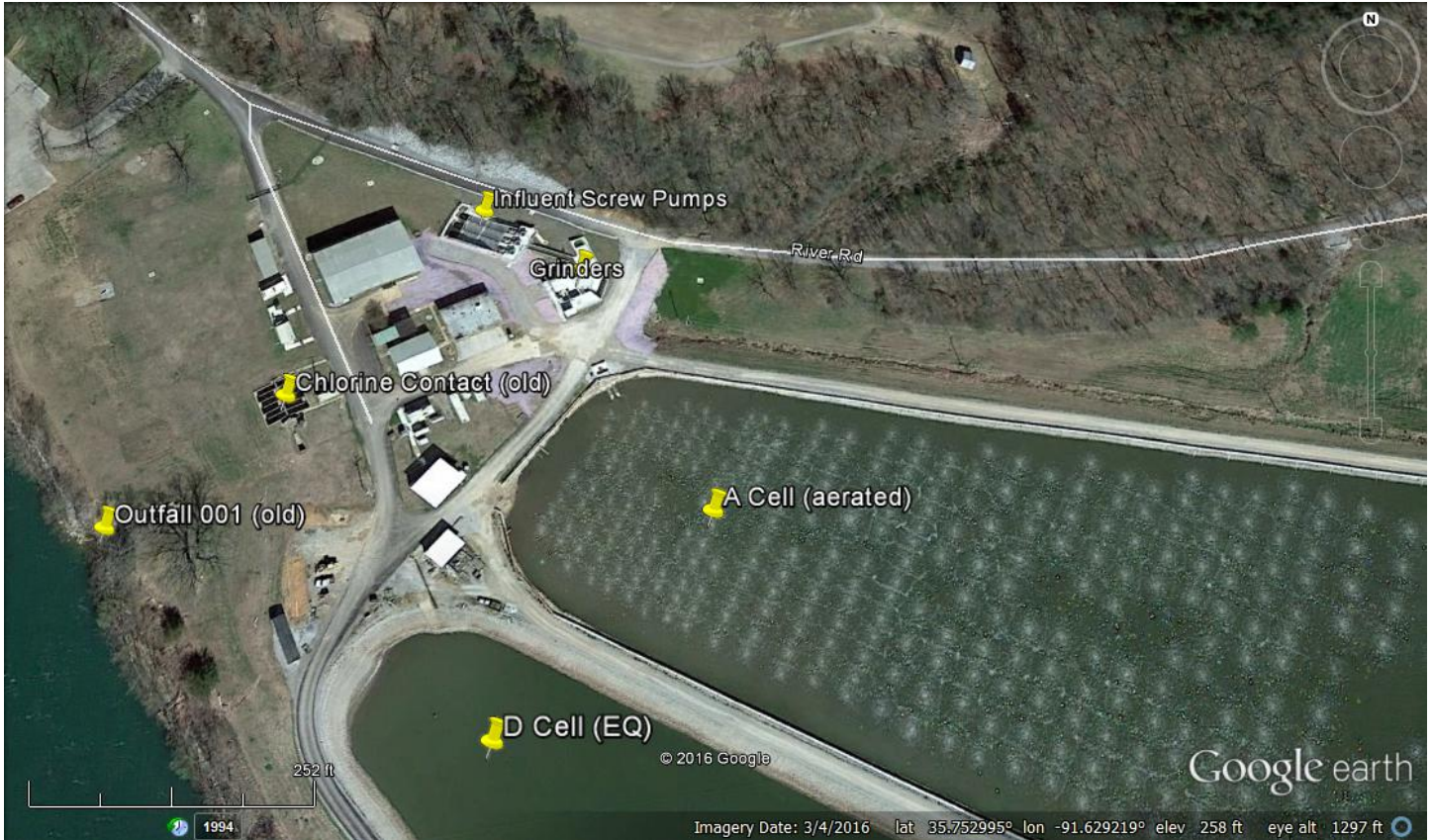
Figure 2. Google Earth image dated March 4, 2016 of headworks of WWTP with major components identified.
