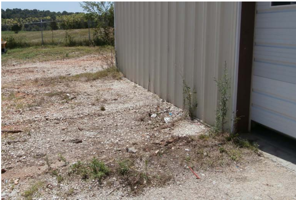
Photo #4 Scrap waste on ground exposed to stormwater – AFTER Scrap metal & bucket removed.
