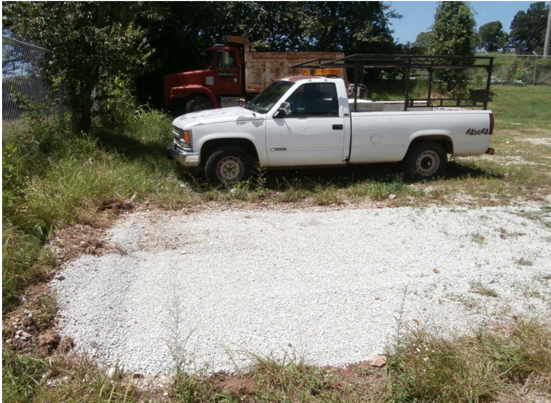
Photo #1 Barrels & buckets unsealed and residuals from spills exposed to stormwater – AFTER Barrels & buckets remove, soil removed, & gravel added.
