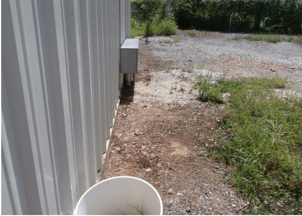
Photo #3 Unsealed/deteriorating bucket and barrel exposed to stormwater – AFTER Barrel & bucket removed, there were no signs of leakage on soil.
