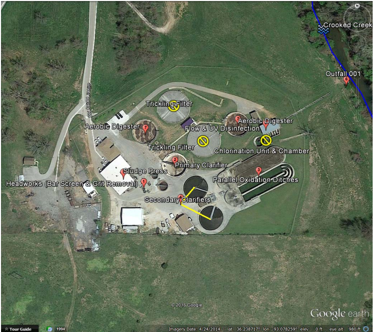
Figure 1. Aerial view of City of Harrison WWTP and associated components (Google Earth: imagery date April 24, 2014). Note trickling filters and chlorination unit/chamber are no longer utilized in the treatment process.
