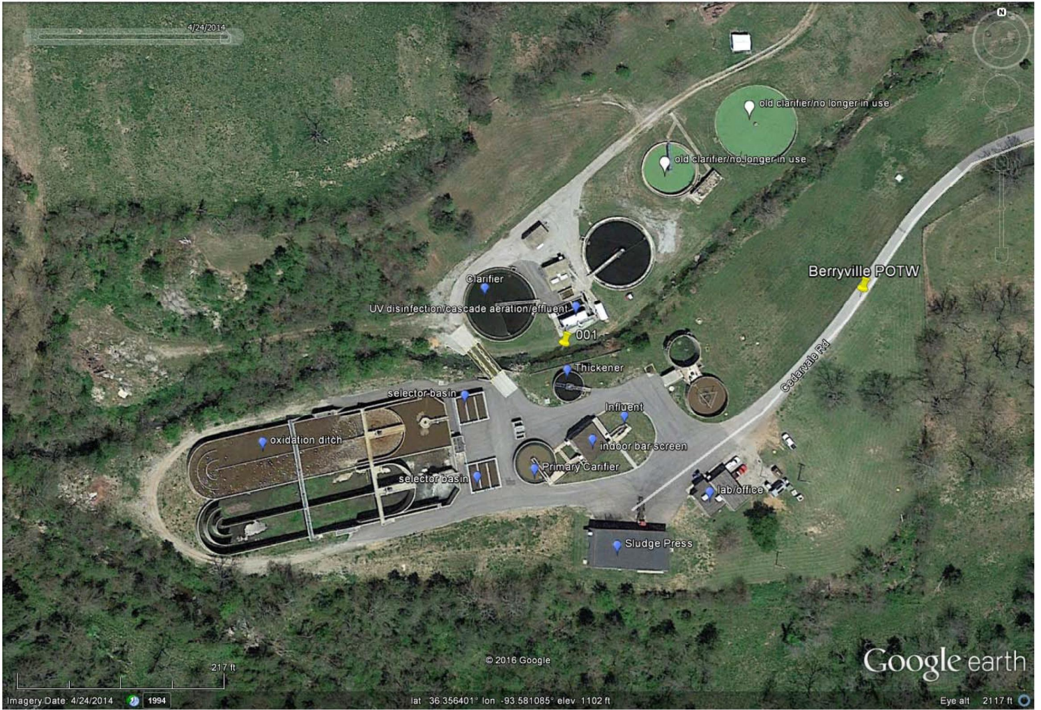
Figure 1. Google Earth image dated April 24, 2014 showing facility overview and major treatment components.
