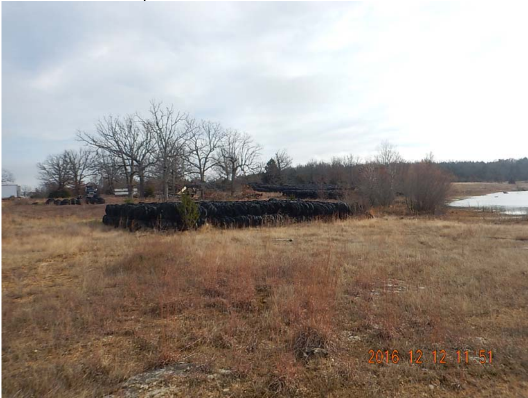
permit 0022-SWTP Photos 5 and 6
