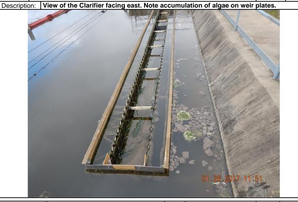
Photographer:Sarah FrasherDate:1/26/2017Time:11:52Witness:Brent WalkerPhoto #:2Description:Close-up view of the Clarifier. Note the accumulation of algae.
