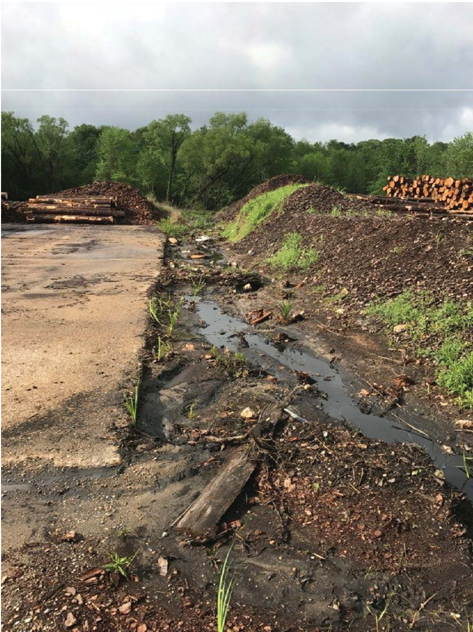
Photograph showing the upper part of the ditch leading to Outfall 008. Vegetation has been established in the lower part of the ditch and starting to grow in the upper portion.
