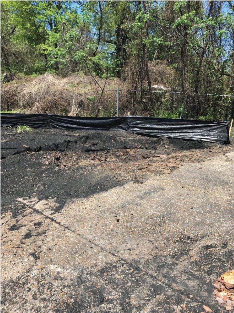
Photograph 1 of silt fence installed down gradient of the kiln ash pile.
