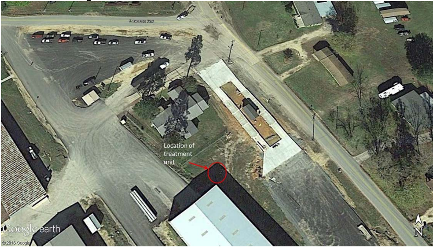
Figure 1. Overview of the location of the ARG550398 treatment unit. Unit serves main office and maintenance building.
