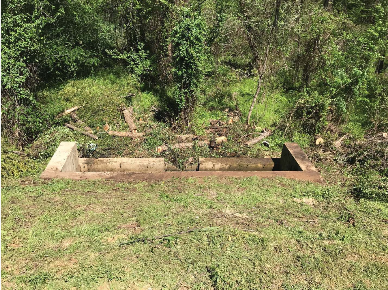
Photograph of Outfall 001 weir.
