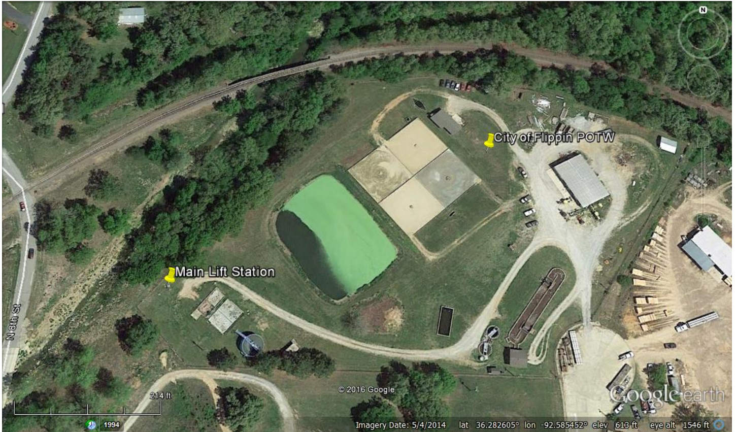
Figure 1. Google Earth image dated May 4, 2014 identifying main lift station at the City of Flippin's POTW.
