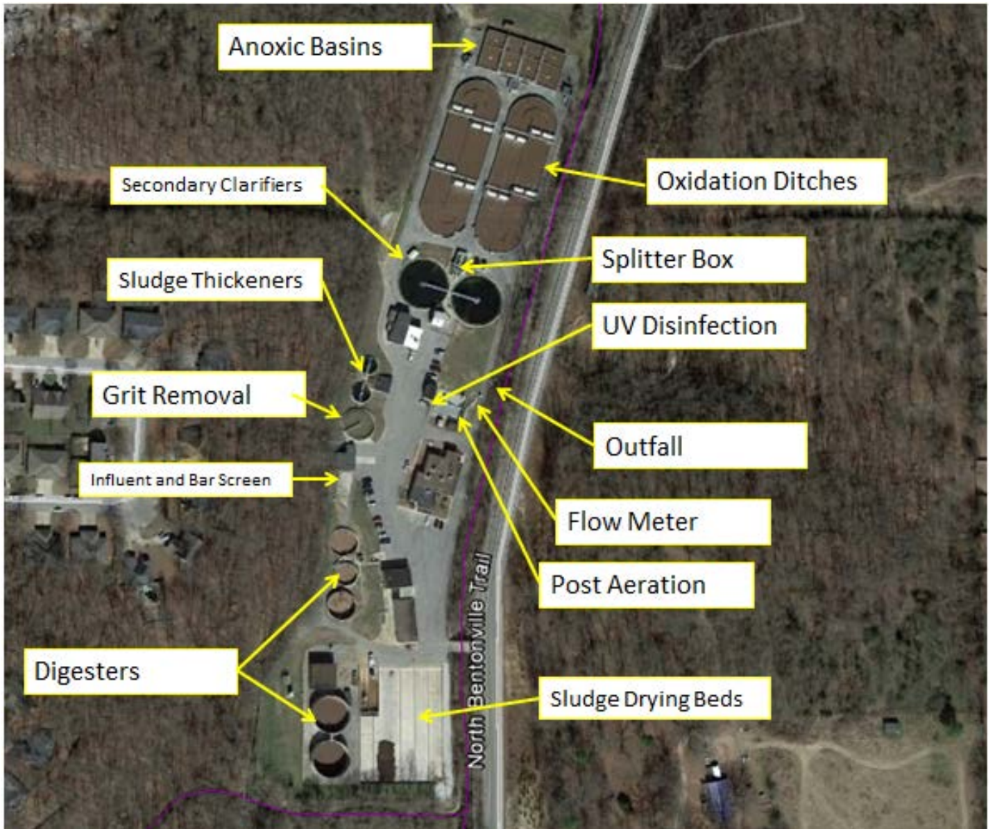
Figure 1: Map of Bentonville's Wastewater Treatment Plant.
