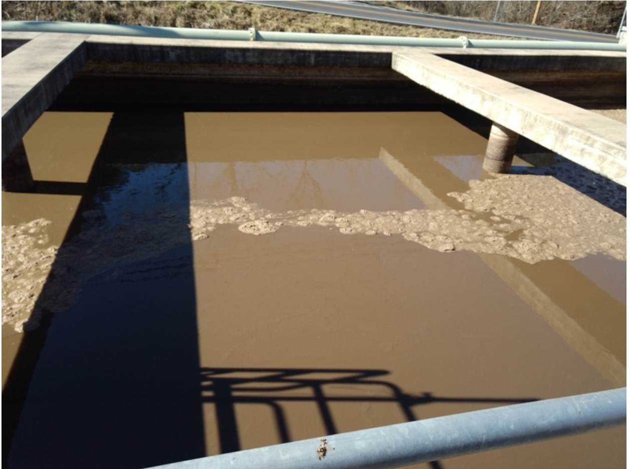
SBR #2 Picture #1 Eureka Springs WWTP
