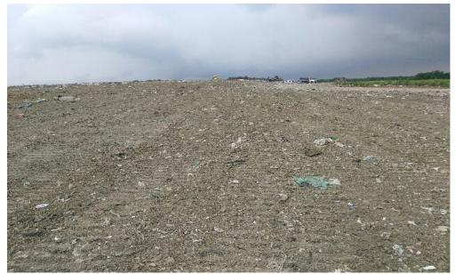
**Corrective Action:** Regulation 411 ( o) was corrected by digging out mattress and replacing void with cover.
