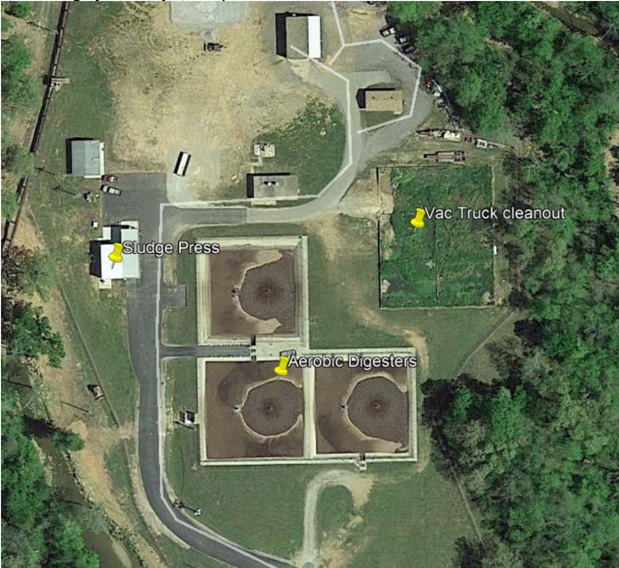
Figure 2. General overview of the northeast part of the WWTP with major components labeled (Google Earth: imagery date May 4, 2014).
