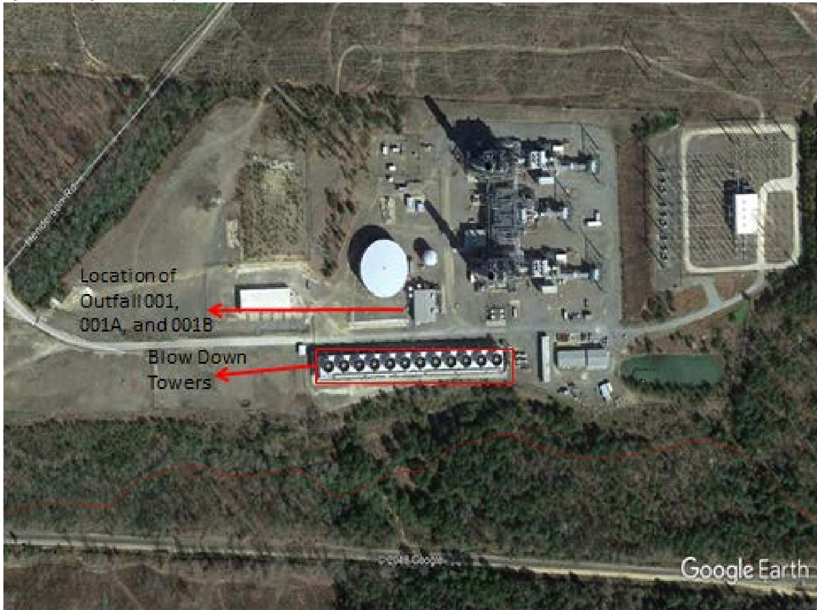
Figure 1: Google Earth image of the facility.
