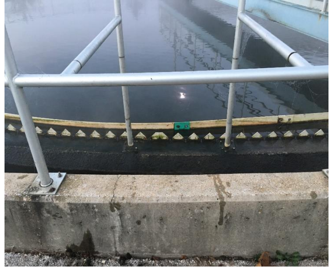
Photo 4 – Baffle repair
