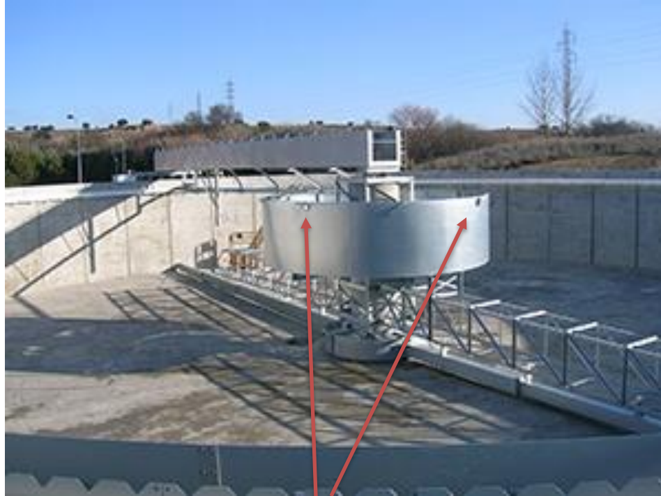
Slots in center ring per manufacturer design
