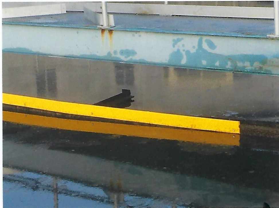
Photo 7 – Temporary repair of skimmer arm on south final clarifier
