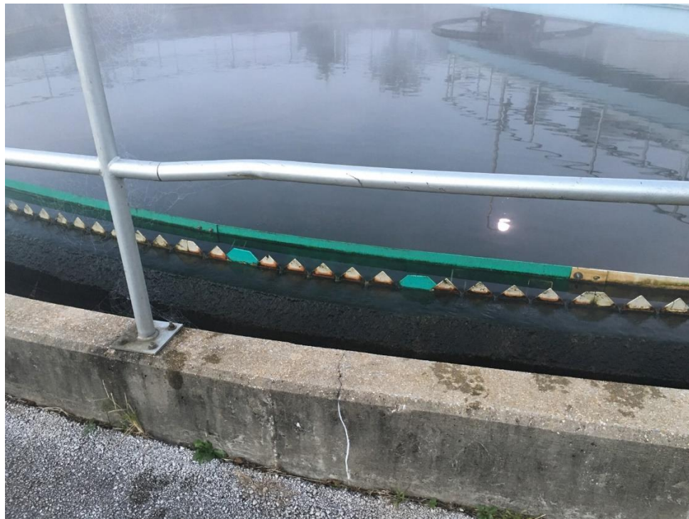
Photo 5 – Weir and baffle repair
