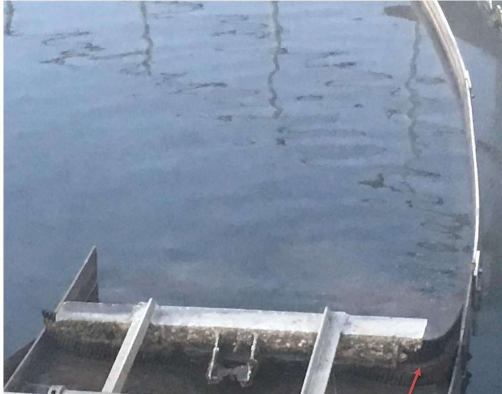
Photo 8 – Skimmer arm with rubber flap connection to edge of outer baffle.
