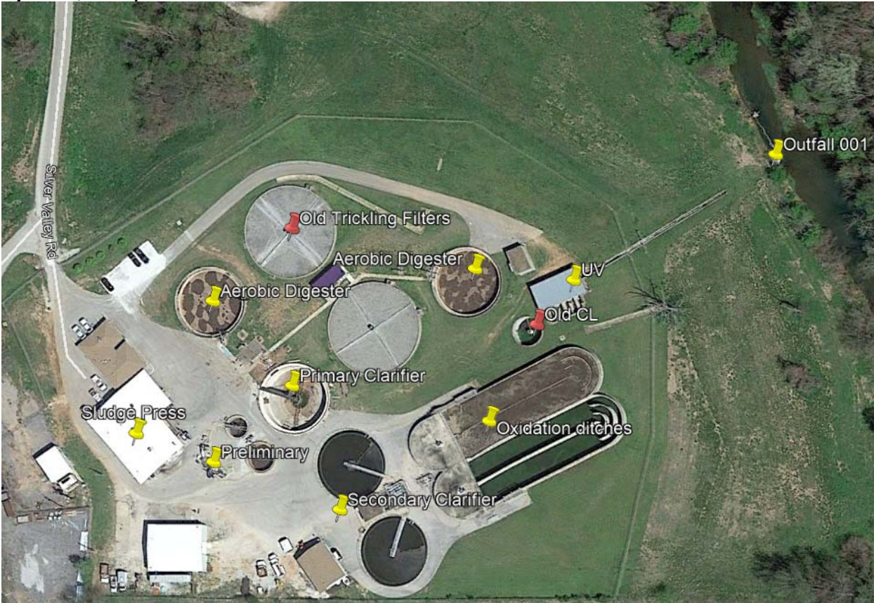
Figure 1. General overview of the WWTP with major components labeled (Google Earth: imagery date April 24, 2014).
