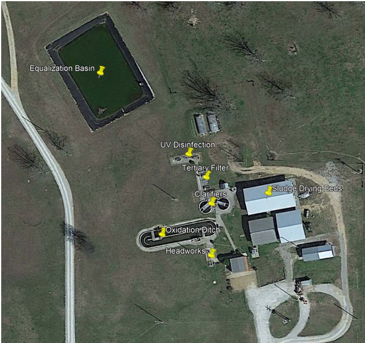
Figure 1. General overview of the WWTP with major components labeled (Google Earth: imagery date March 21, 2016).
