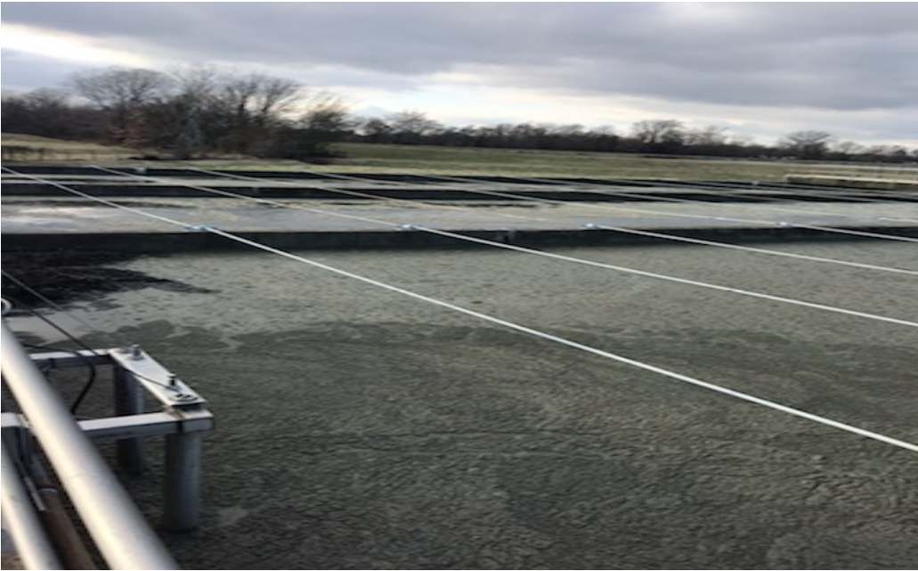
WWTP-Oxidation Ditch (Photo 2)
