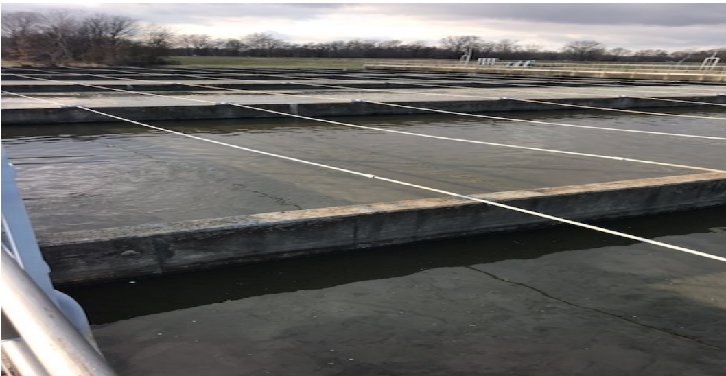
WWTP-Oxidation Ditch (Photo 1)
