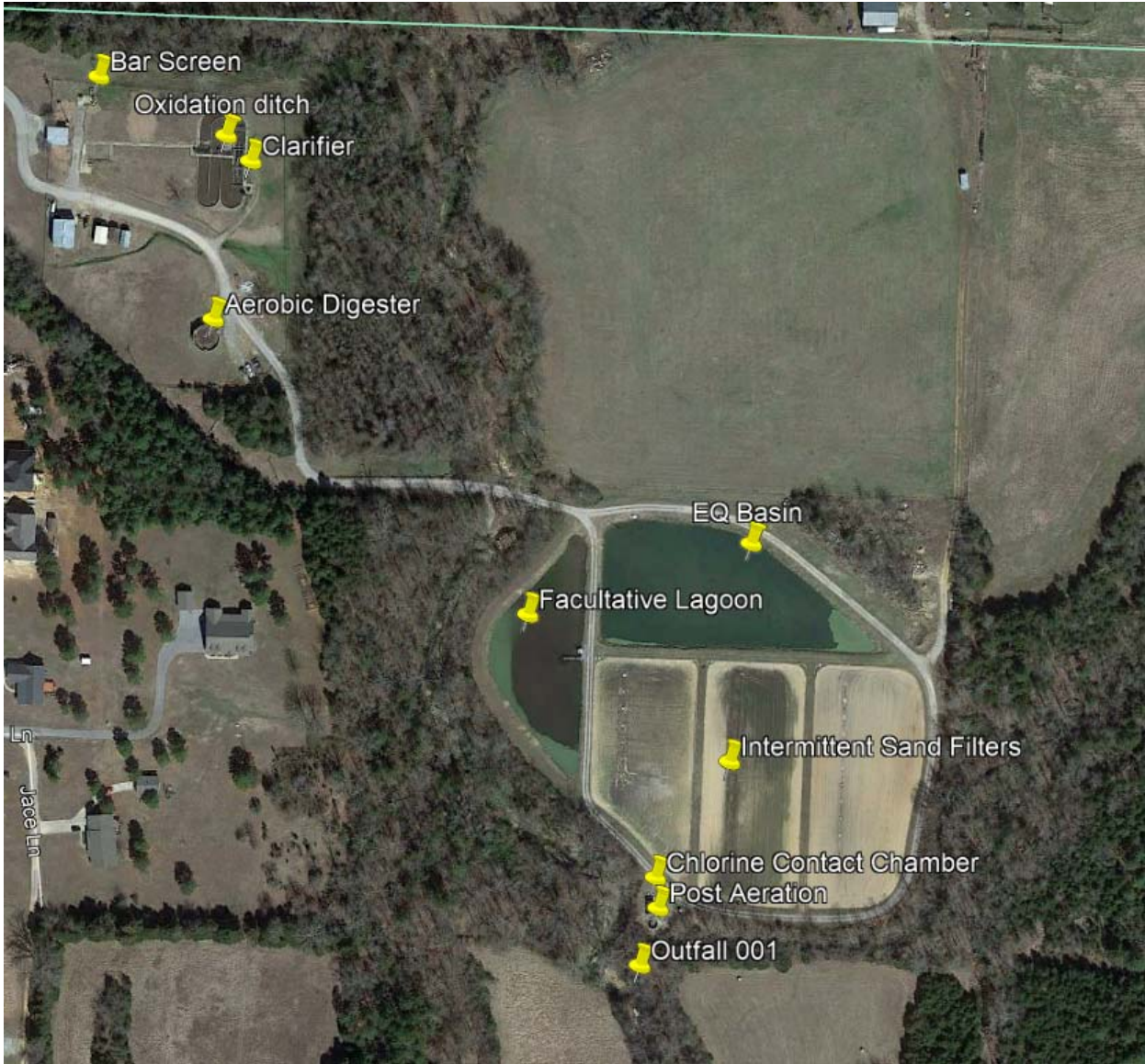
Figure 1. General overview of the site with major WWTP components labeled (Google Earth: imagery date March 4, 2016).
