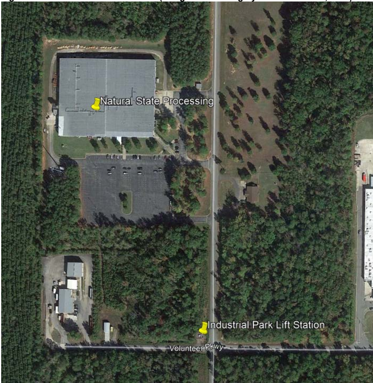
Figure 1. General overview of the site (Google Earth: imagery date October 16, 2014).
