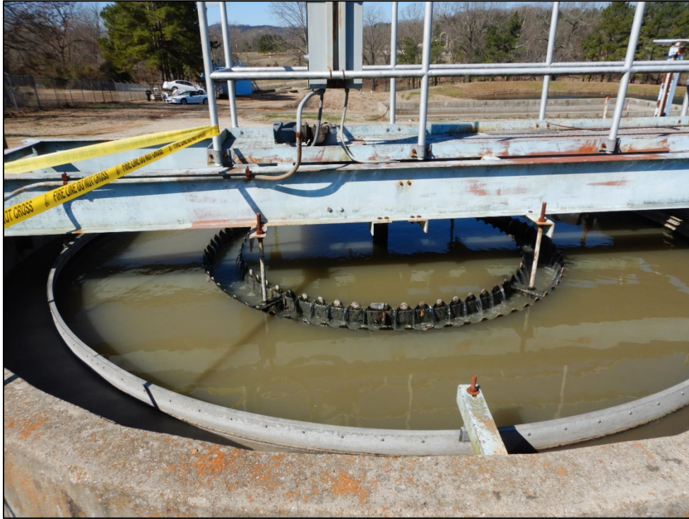
Photograph 5. Secondary clarifier No. 1.
