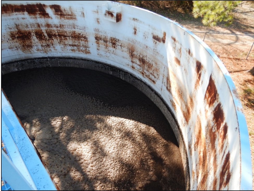
Photograph 11. View inside digester.
