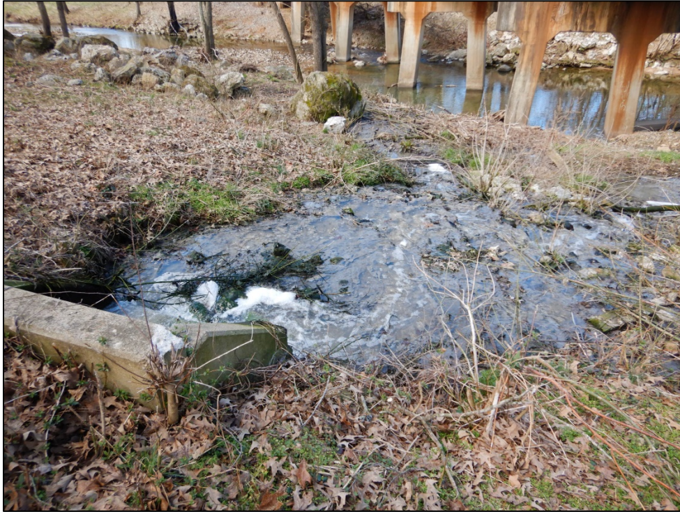
Photograph 9. Outfall and receiving waterbody.
