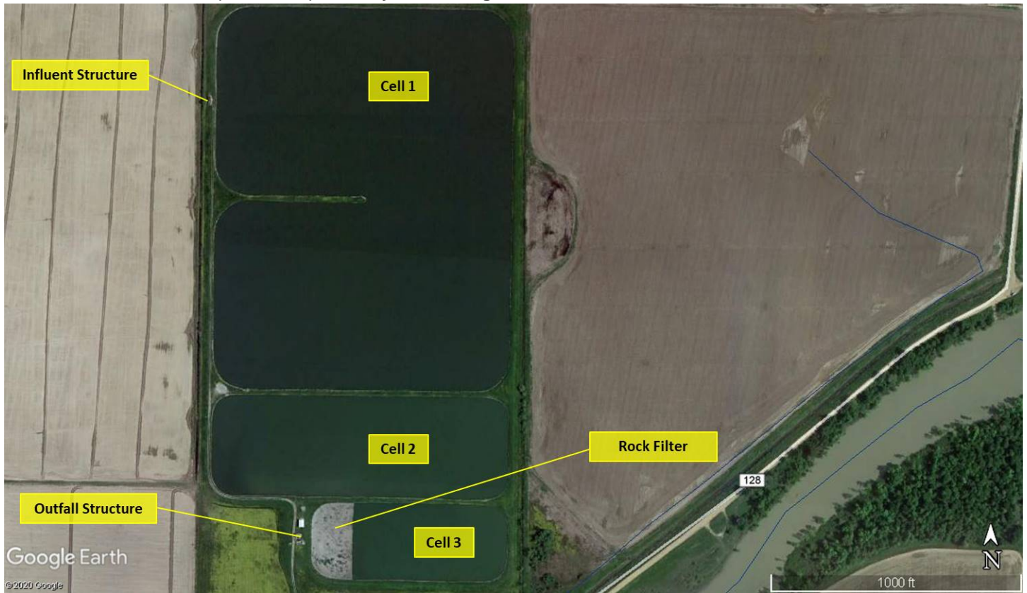
Figure 1. Google Earth image of the City of Corning with labels for the different areas of treatment.
