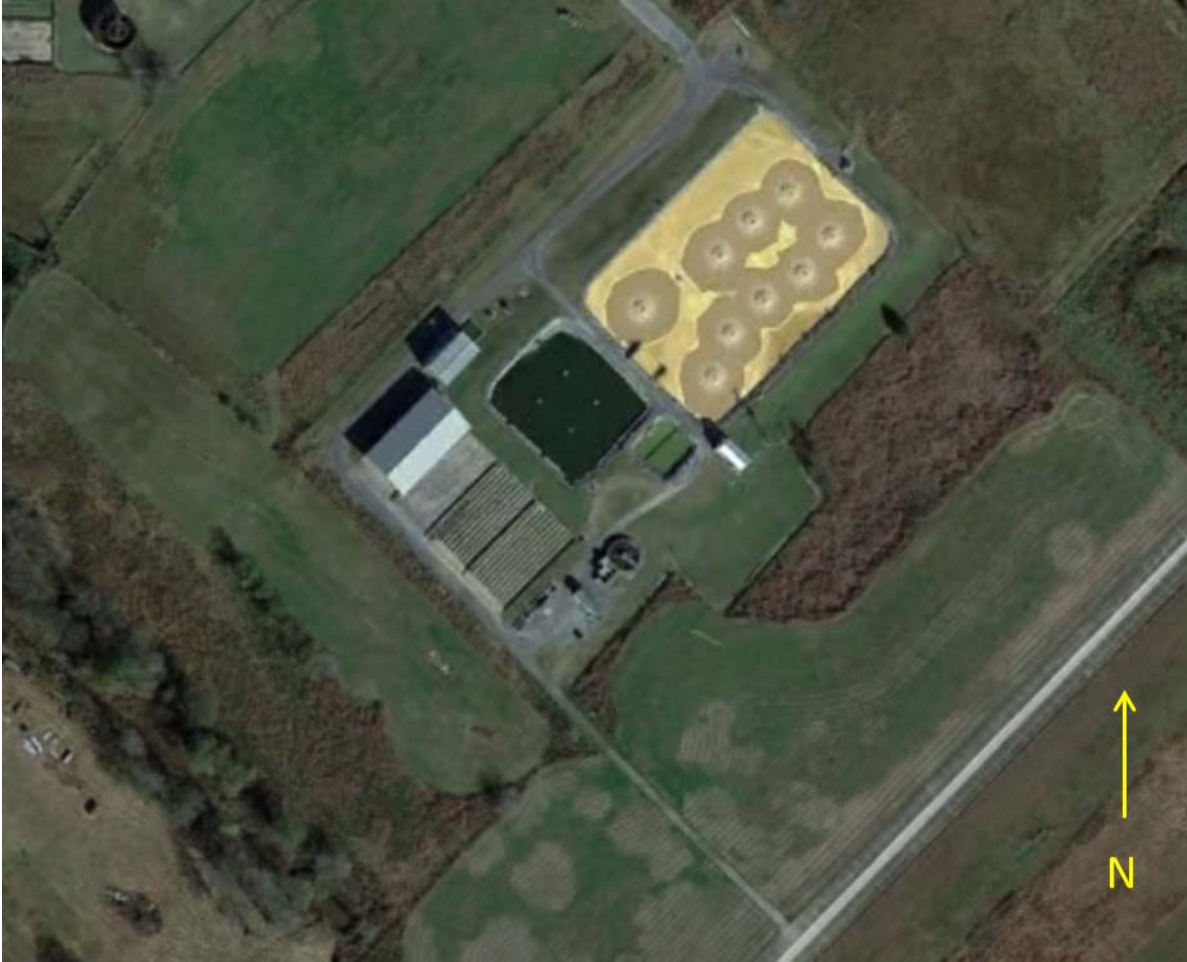
Figure 1: Google Earth image of site, imagery date of 11/15/2020.
