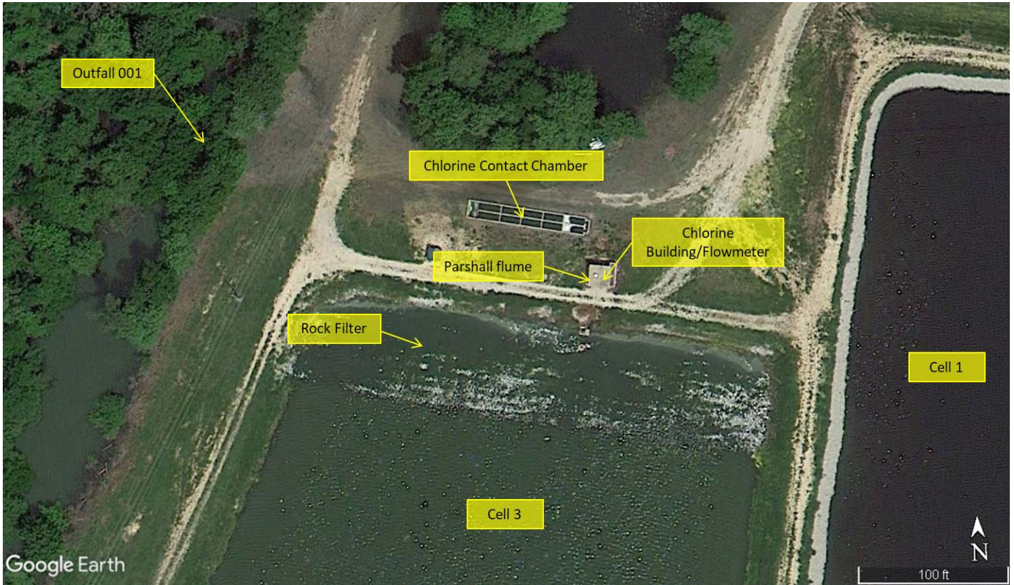
Figure 2. Google Earth image zoomed into the City of Pocahontas WWTP with labels for the specific areas of treatment.
