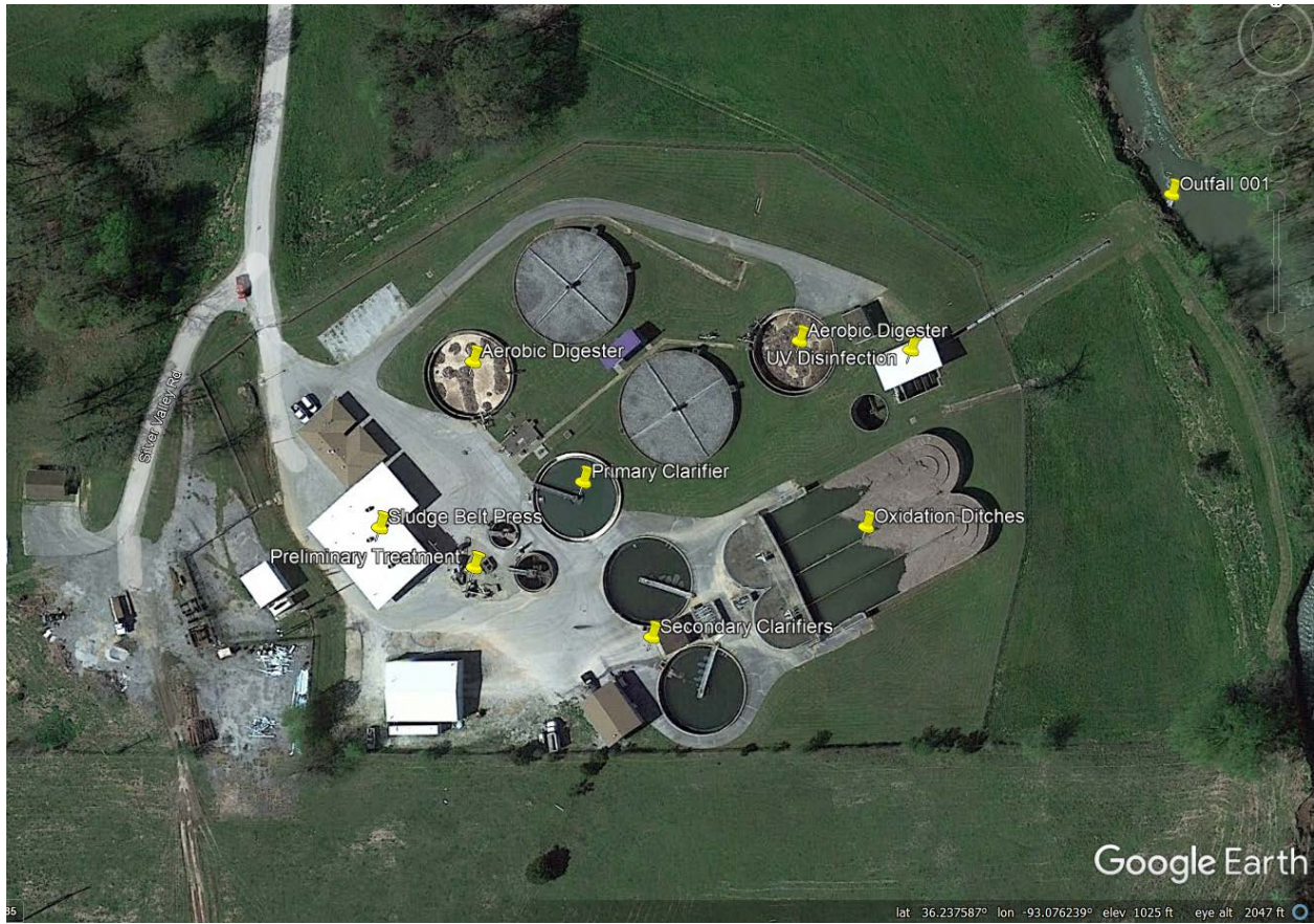
Figure 1. Google Earth image dated April 4, 2019 of the POTW and its major components and Outfall 001.
