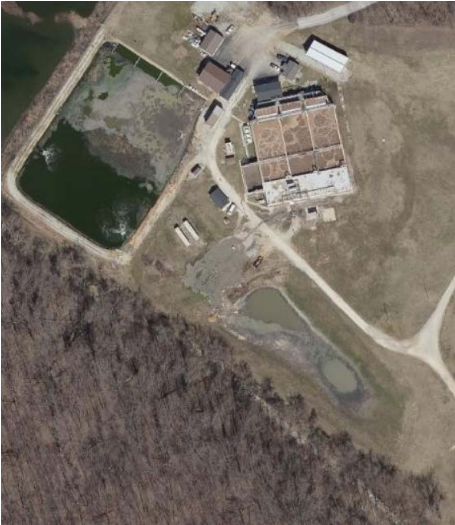
Attachment 3: Satellite image showing overflow from the MBR to the storage pond.
