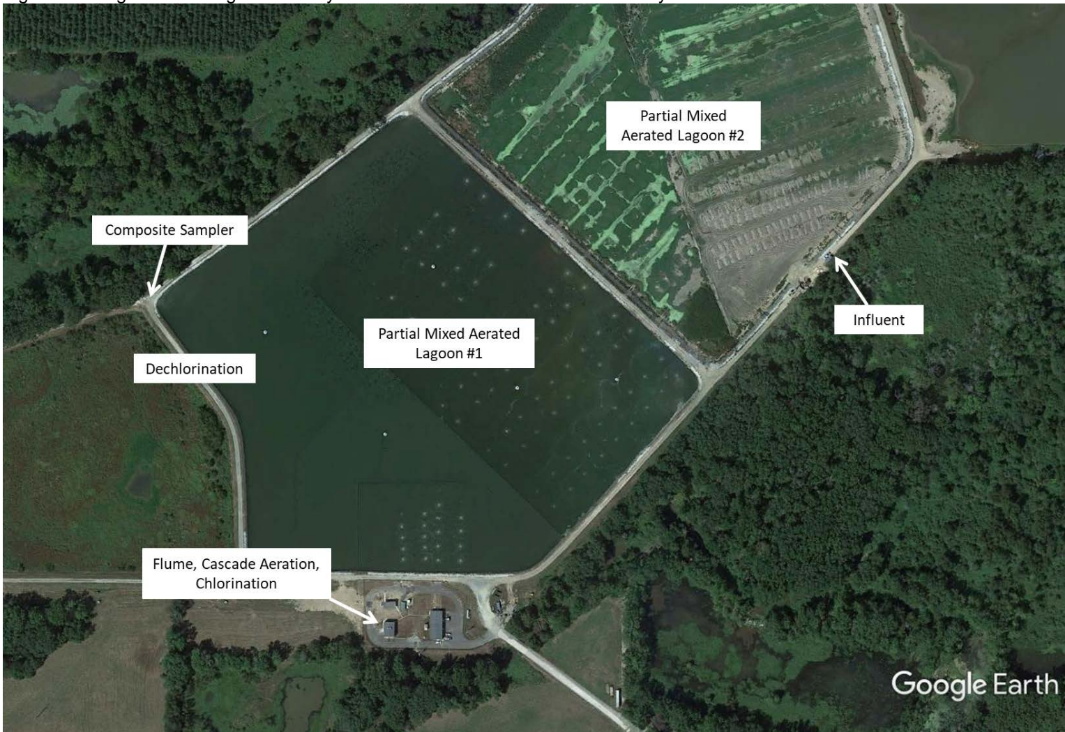
Figure 1: Google Earth image of the City of Malvern wastewater treatment facility.
