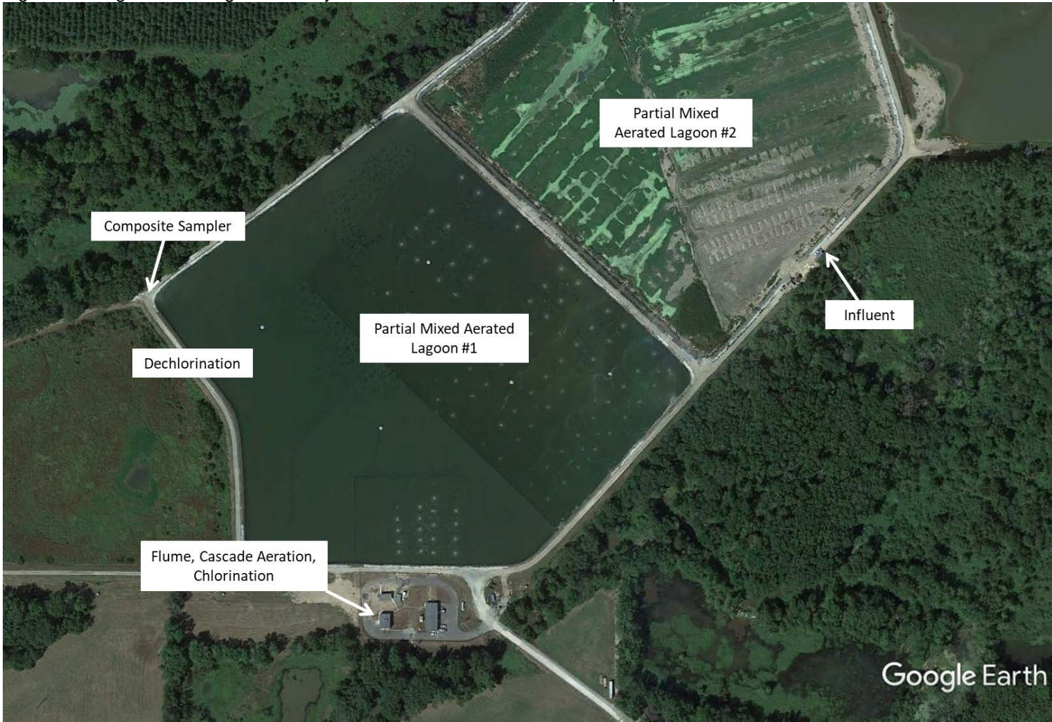
Figure 1: Google Earth image of the City of Malvern wastewater treatment plant.
