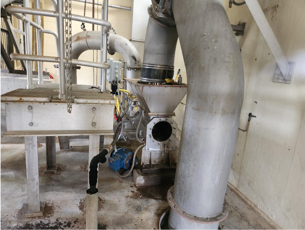
Photo 1 Compactor missing gearbox
