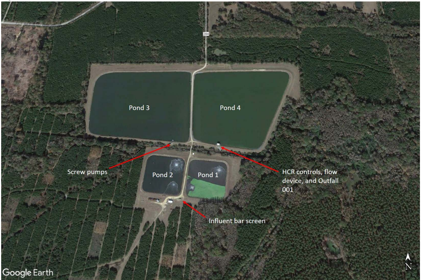
Figure 1. Overview of the Monticello East Plant.
