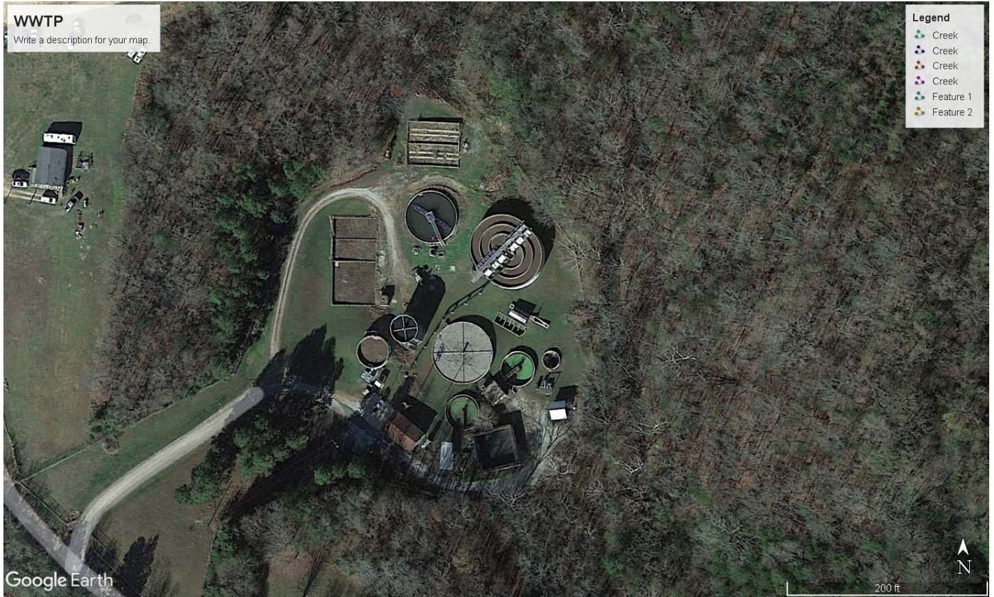
Figure 1. Google Earth image of treatment facility.
