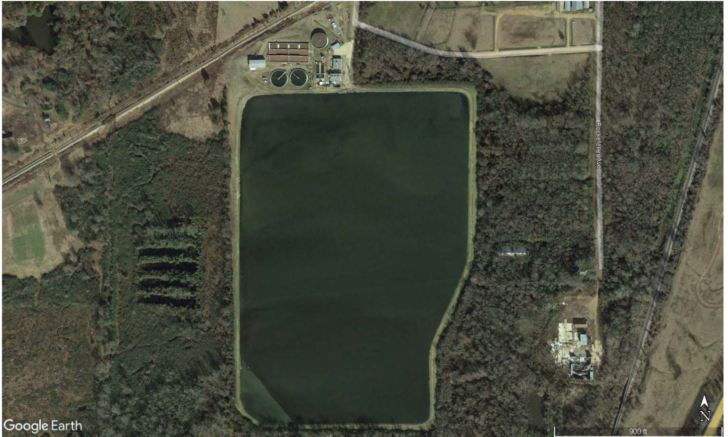
Figure 1. Overview of City of De Queen wastewater treatment plant with the equalization basin and treatment components.
