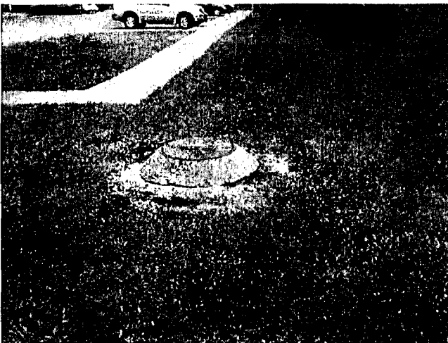
Figure 4: Manhole ring grout separated from cone section near Park Avenue; likely damaged by mowing machinery. Displacement will allow inflow. Repairs are planned.
