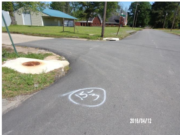
Figure 8 – Example of covered manhole
