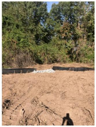
Storm Water Catch Basin was under construction as of October 17<sup>th</sup>. Note it is protected by silt fence to prevent silt from entering the storm drain.
