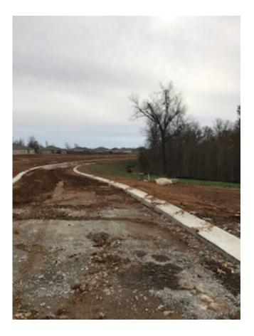
Storm drain outflow is temporarily protected with native rocks to disburse the water and prevent erosion as it enters the vegetated drainage basin.
