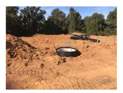
Curbs were installed the week of 12-1-17 all potential runoff from the road bed is being contained within the curbs. Storm drains are currently closed to prevent water for entering. You can see on the down slope that the entire perimeter has been protected by Silt Fence as well as a buffer of fresh grass. The storm water plan calls for the disbursement and release of runoff that is captured in the storm drain system onto highly vegetated areas.
