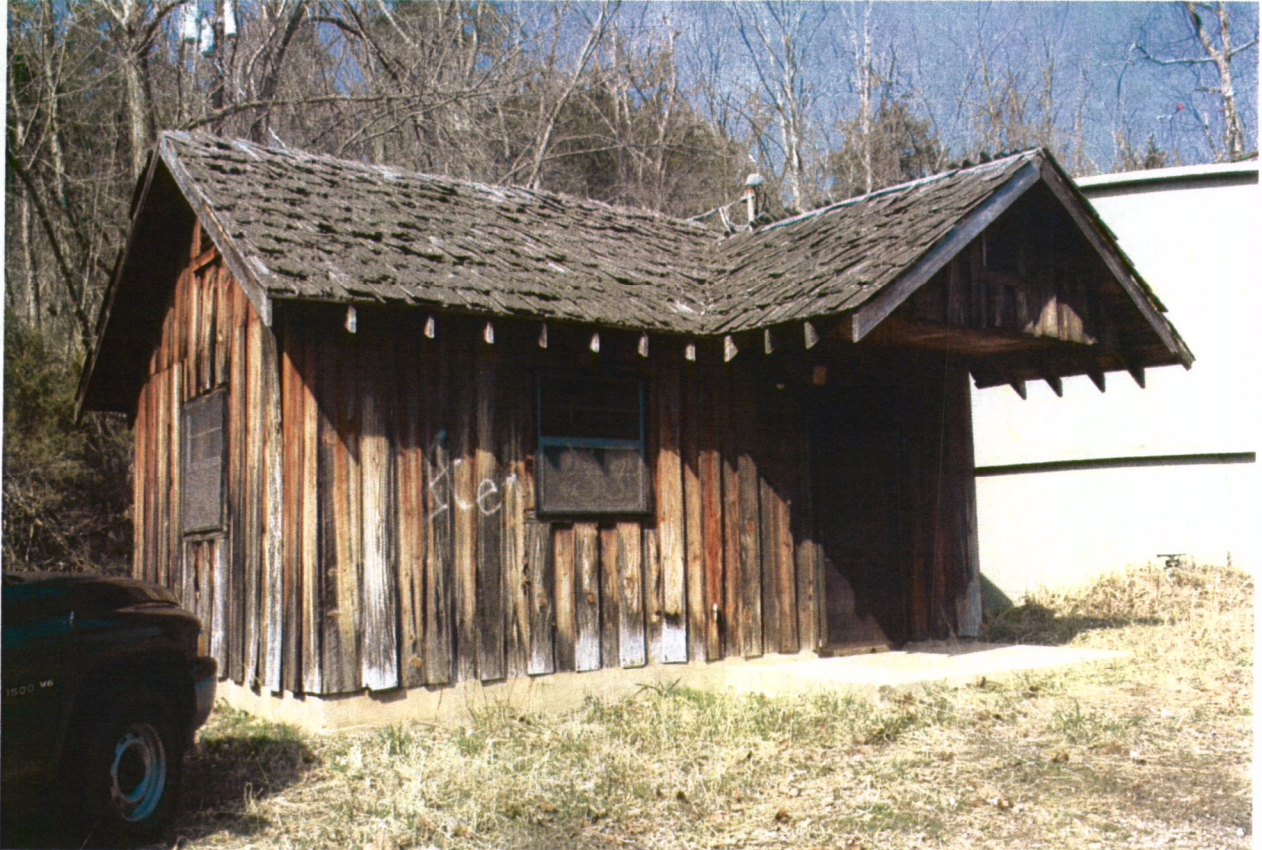
Figure 3.23 Equipment Building Photo
