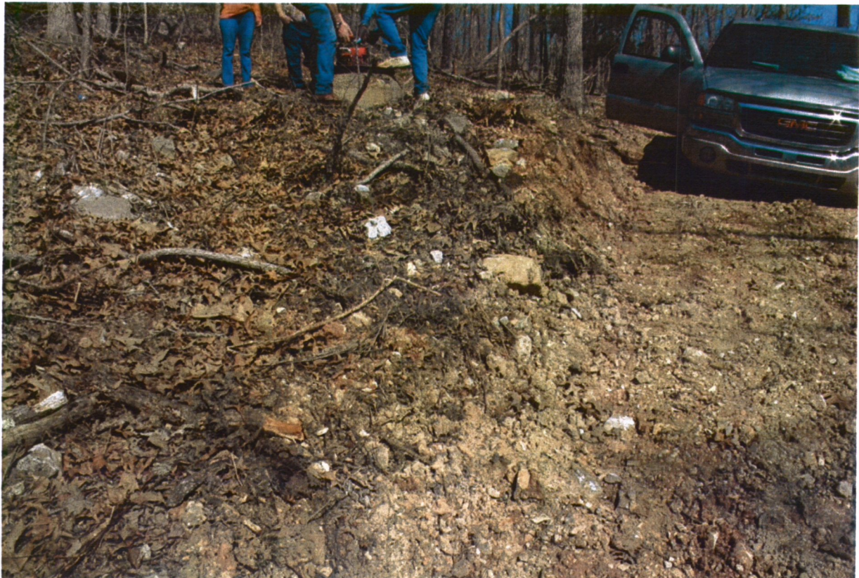
Figure 3.10 Debris Below Manhole 1-D (ARWA MH #34)
