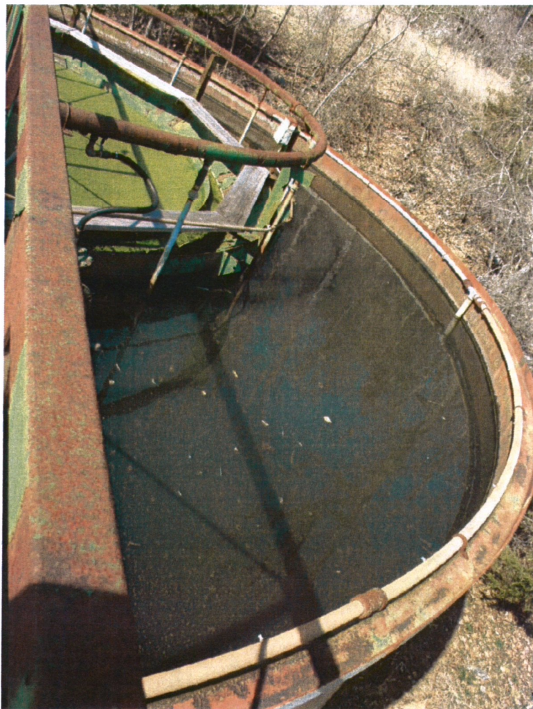
Figure 3.38 Aeration Piping and Spray Nozzles
