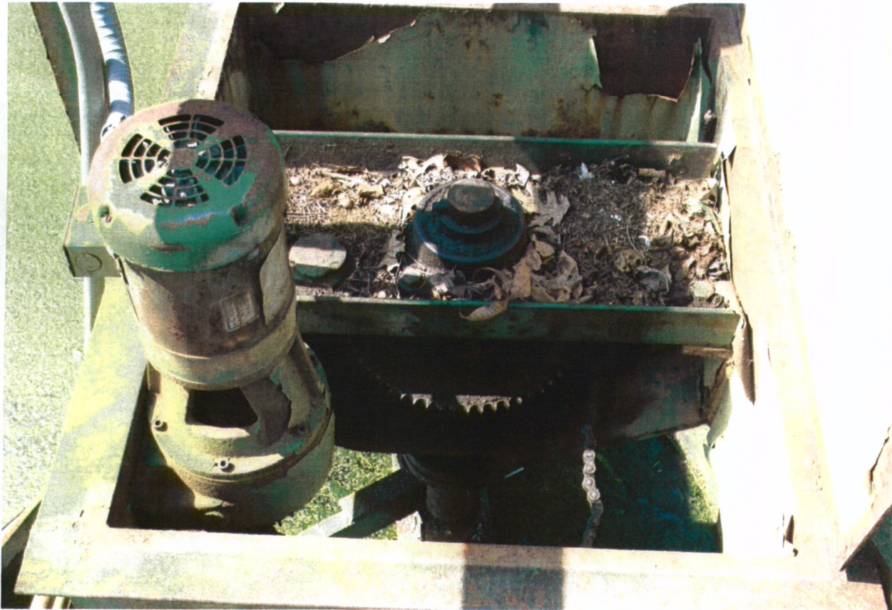
Figure 3.41 Skimmer Arm Motor, Chain, and Gear
