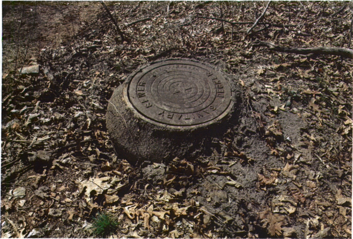
Figure 3.9 Manhole 1-D (ARWA MH #34)
