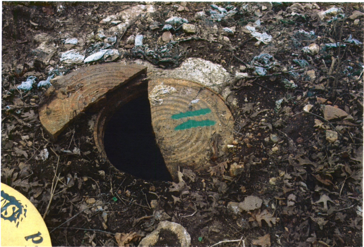
Figure 3.12 Manhole 4-Q (ARWA MH #11)
