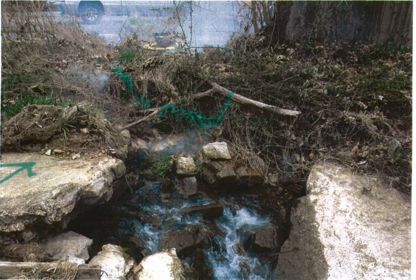
Figure 3.17 Smoke Escaping Near Manhole 4-K (ARWA MH #17)
