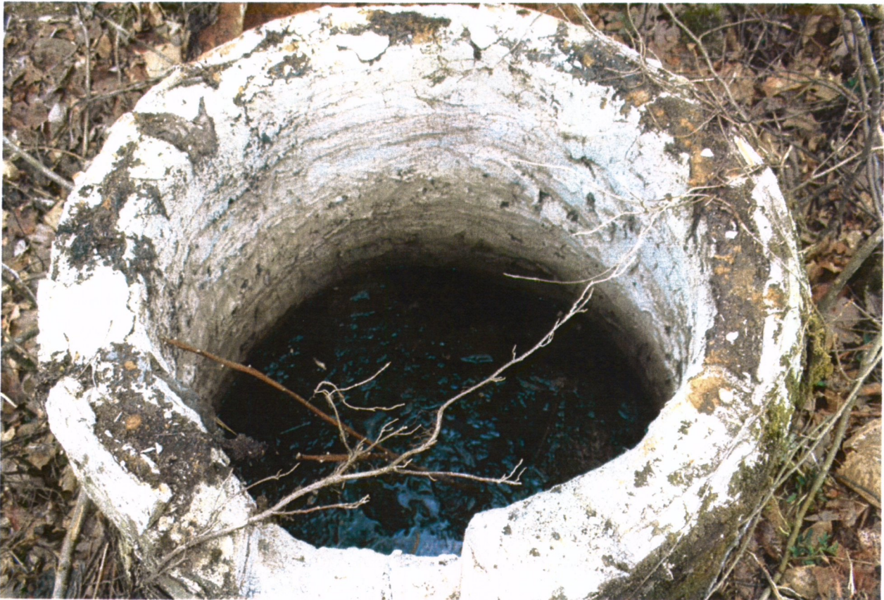
Figure 3.15 Manhole 4-O (ARWA MH #13)
