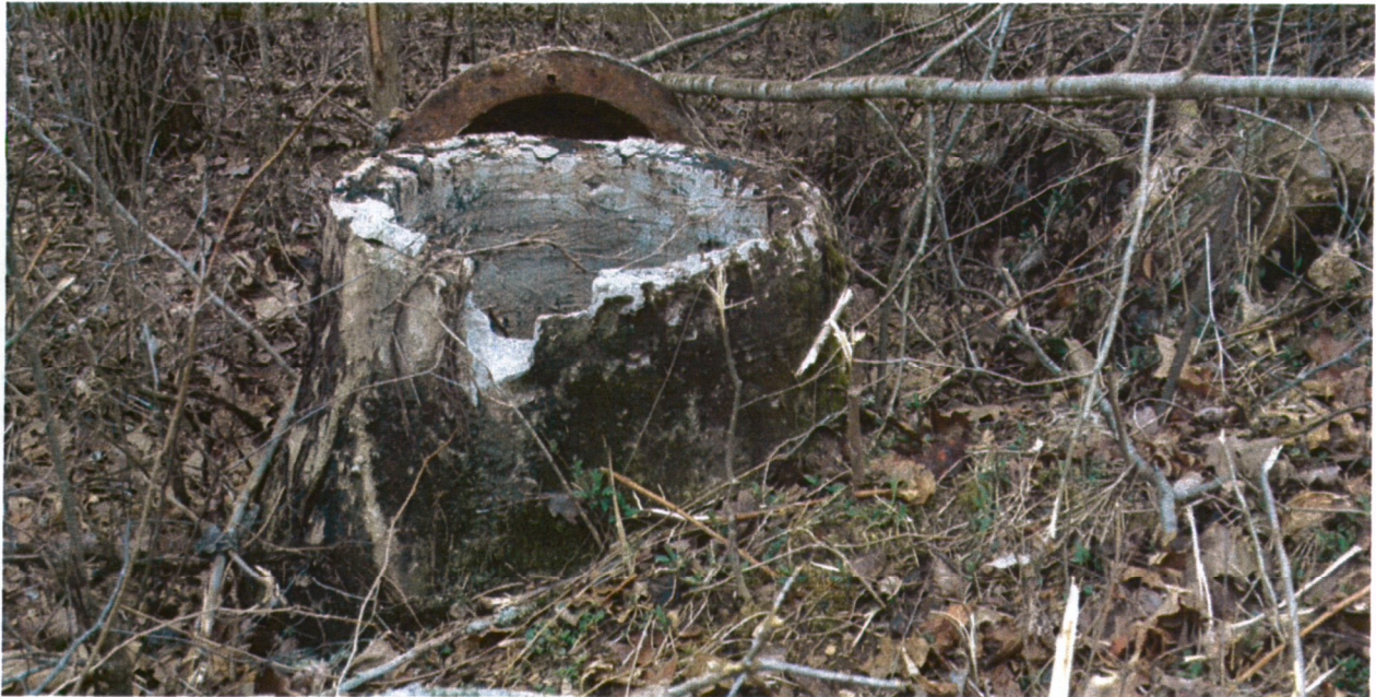
Figure 3.14 Manhole 4-O (ARWA MH #13)
