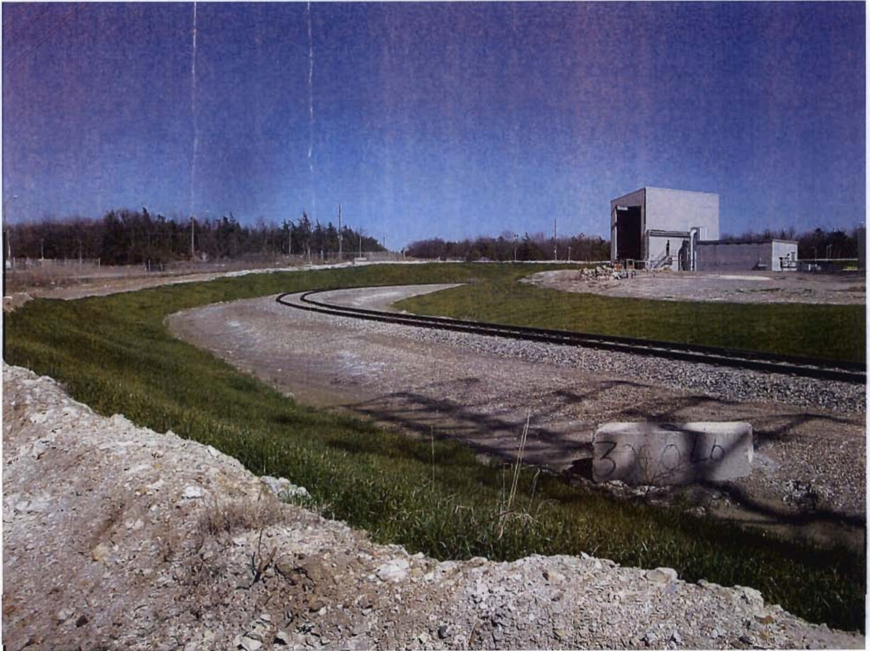
Figure 10 W side of rail unloading
