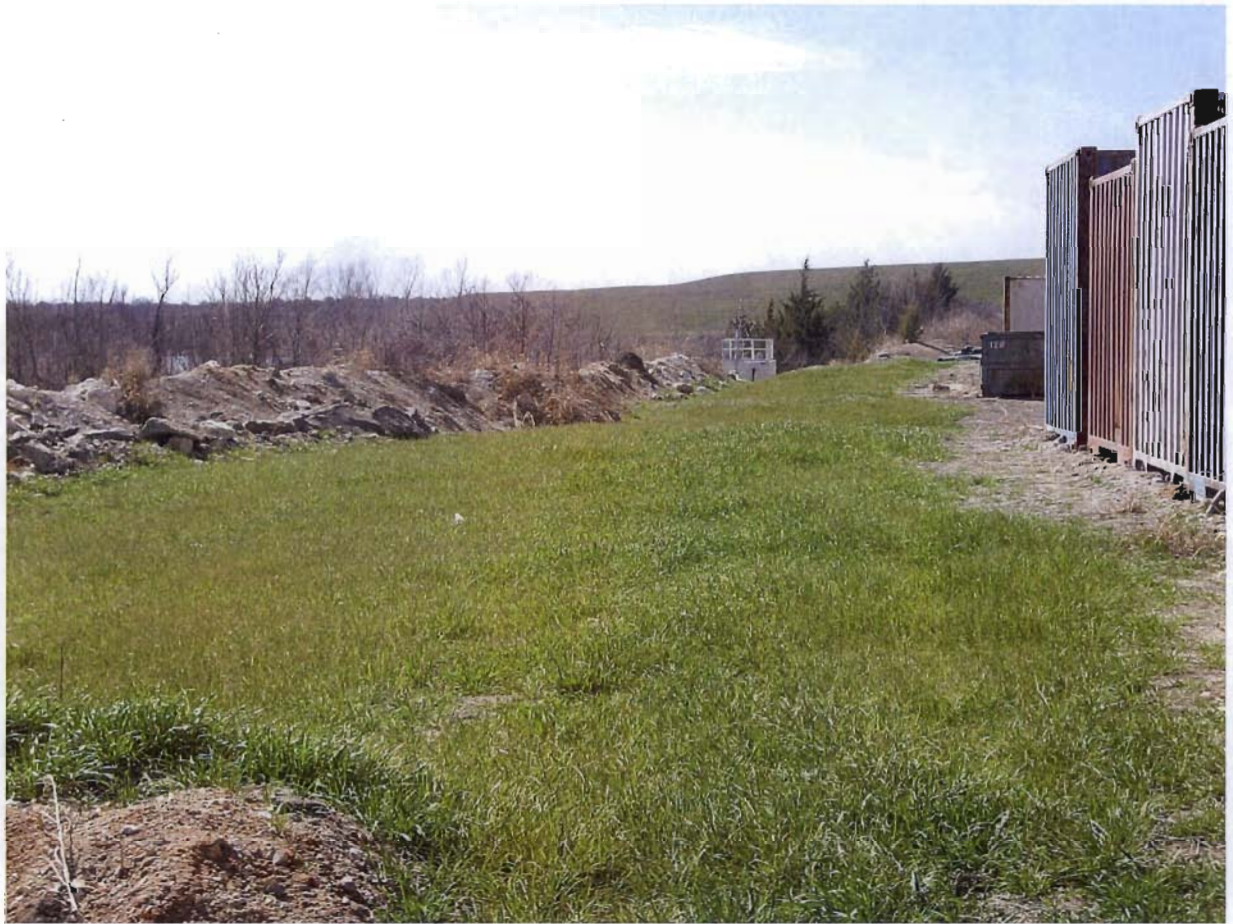
Figure 16 slope N of pond near WWTP
