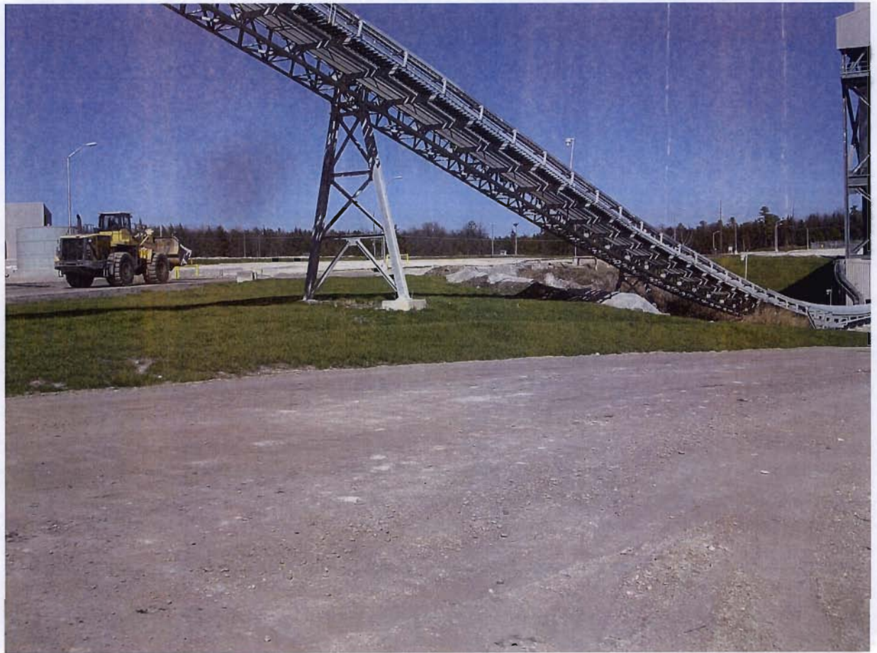
Figure 6 Under raw material belt
