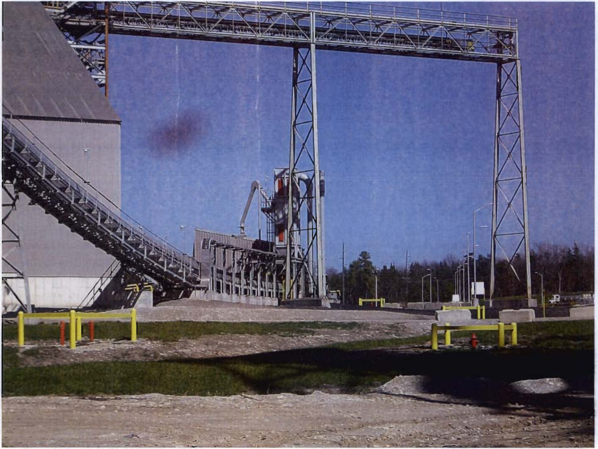
Figure 7 S side of Coal Apron Feeder
