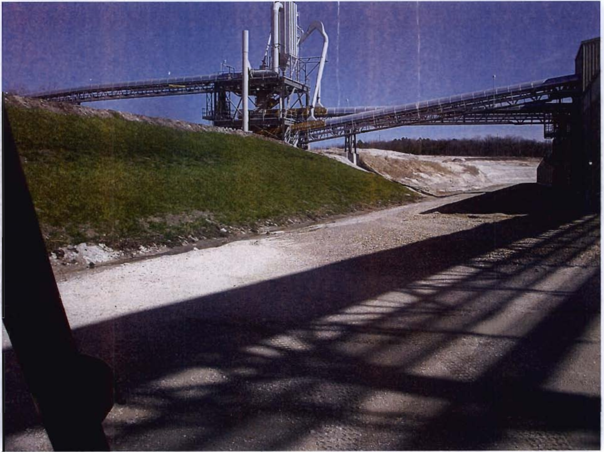
Figure 5 N side of MSB Building
