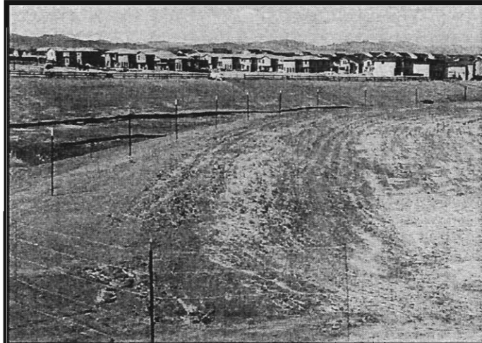
A temporary diversion dike can be stabilized with straw mulching.
