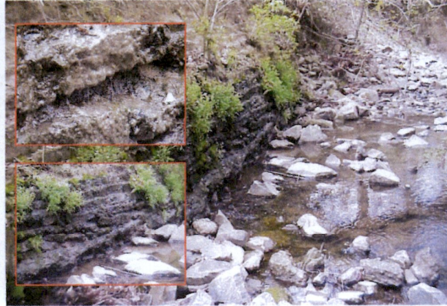
Leaking Sewer Collection Line
