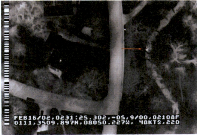
Infrared Aerial Photograph of a Leaking Sanitary Sewer Line
