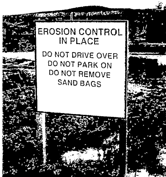
Figure 4. Use signage to help educate construction staff.
