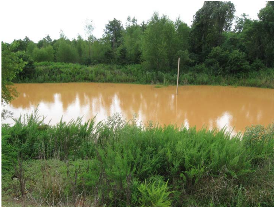
Photo 4. Class 4 stormwater pond, looking south.
