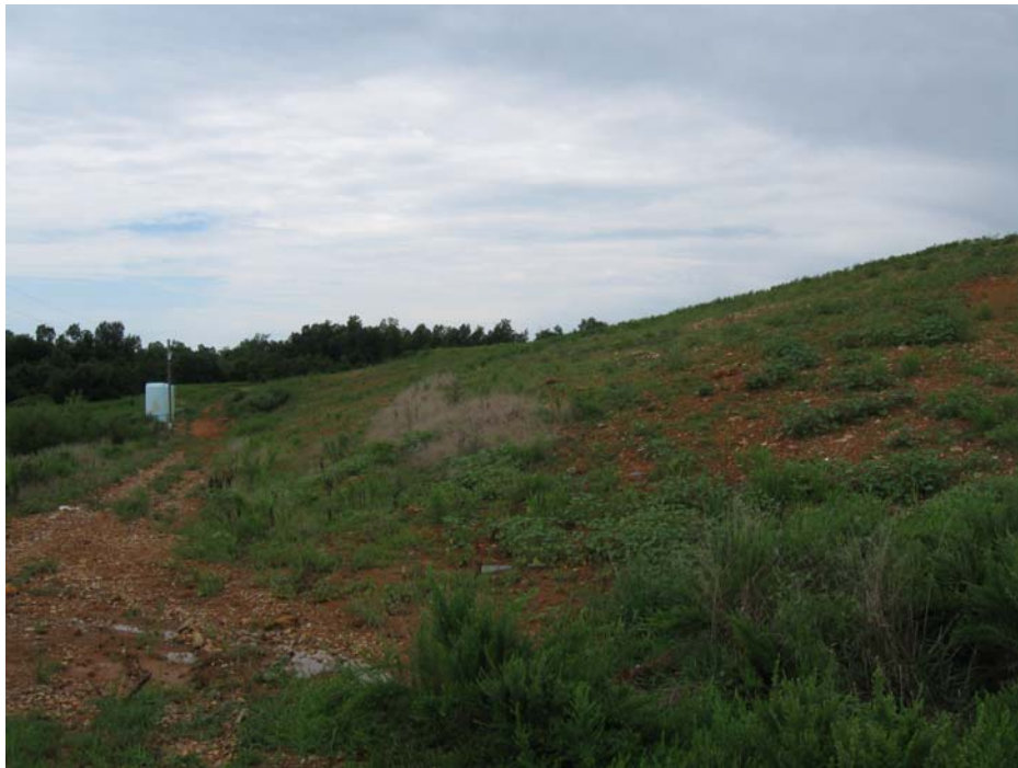
Photo 2. Class 4 Landfill, looking west at Cells 5 and 6.
