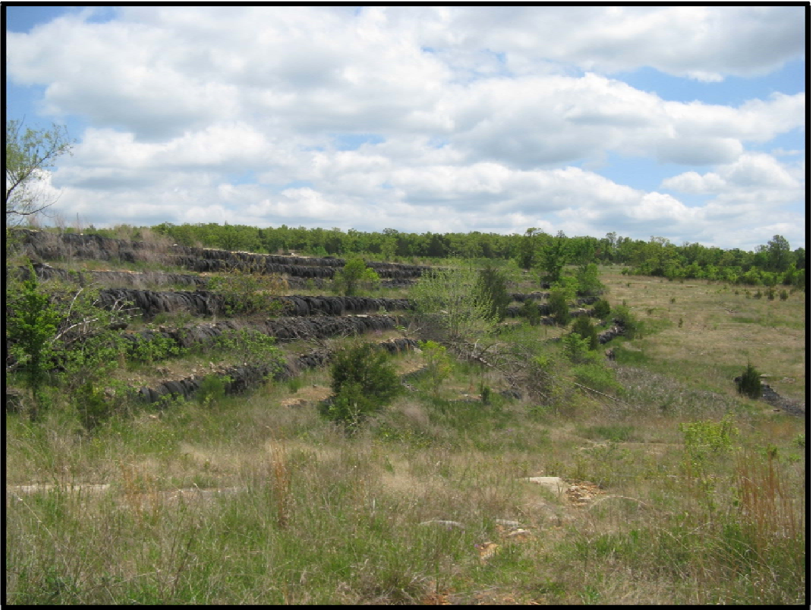
Photo 7: Looking southeast at western slope of dam; middle bench is at upper surface of exposed baled tires.
