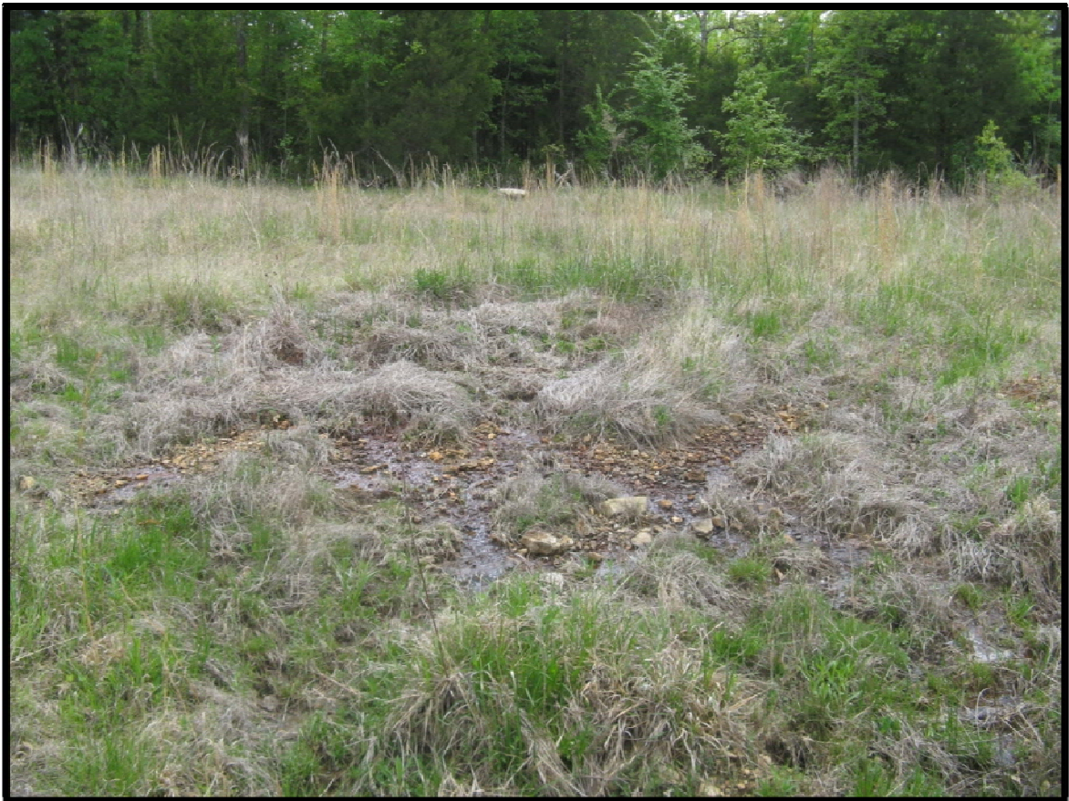
Photo 6: Seepage flowing west from toe of slope.
