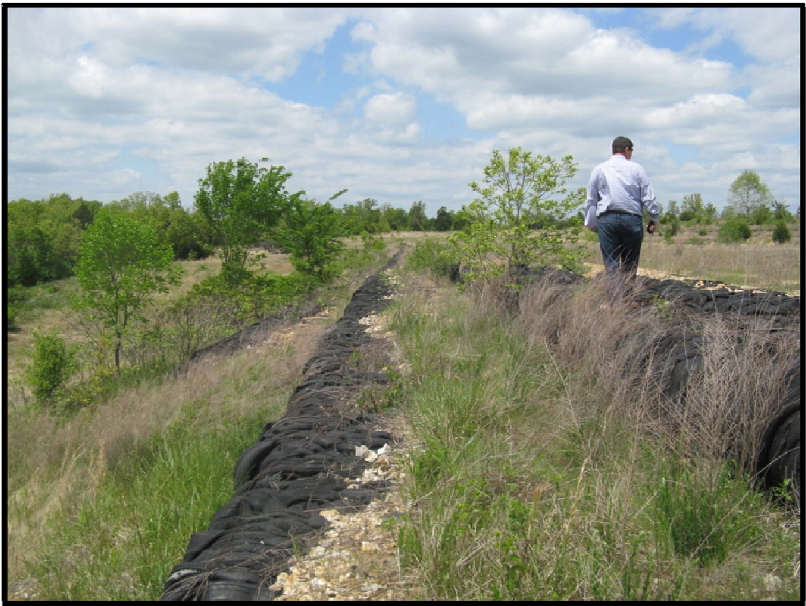
Photo 3: Looking northwest at western edge of middle bench; note exposed baled tires.
