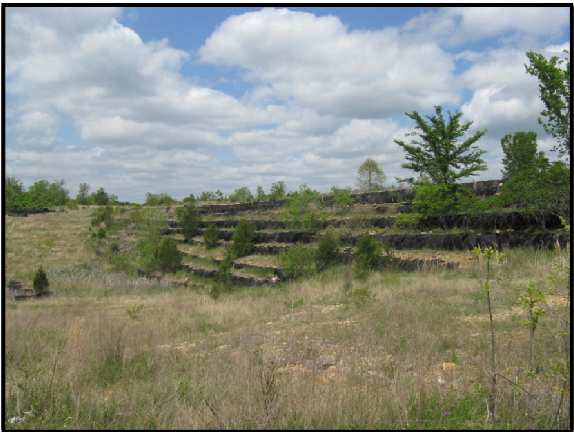
Photo 4: Looking north at western edge of middle bench on right and lower bench on the left; note exposed baled tires.
