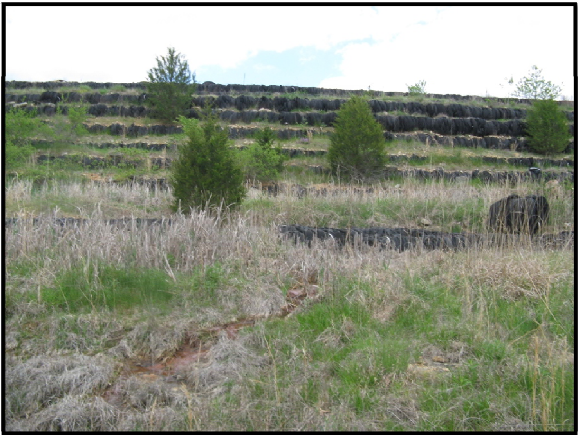
Photo 5: Looking east at western slope of dam; middle bench is at top of photo and lower bench is in middle of photo; note seepage (orange staining) in foreground.
