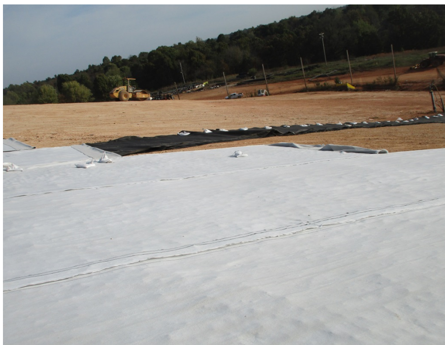
Photo 4 – GCL is placed over Geocomposite Gas Vent
