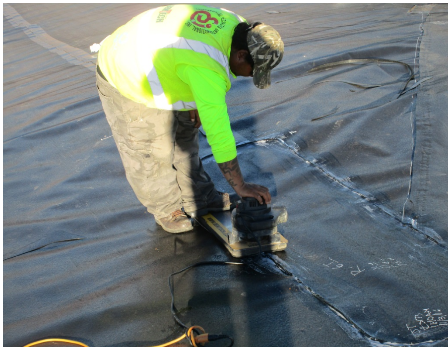
Photo 15 – Vacuum Testing Extrusion Welded Repairs
