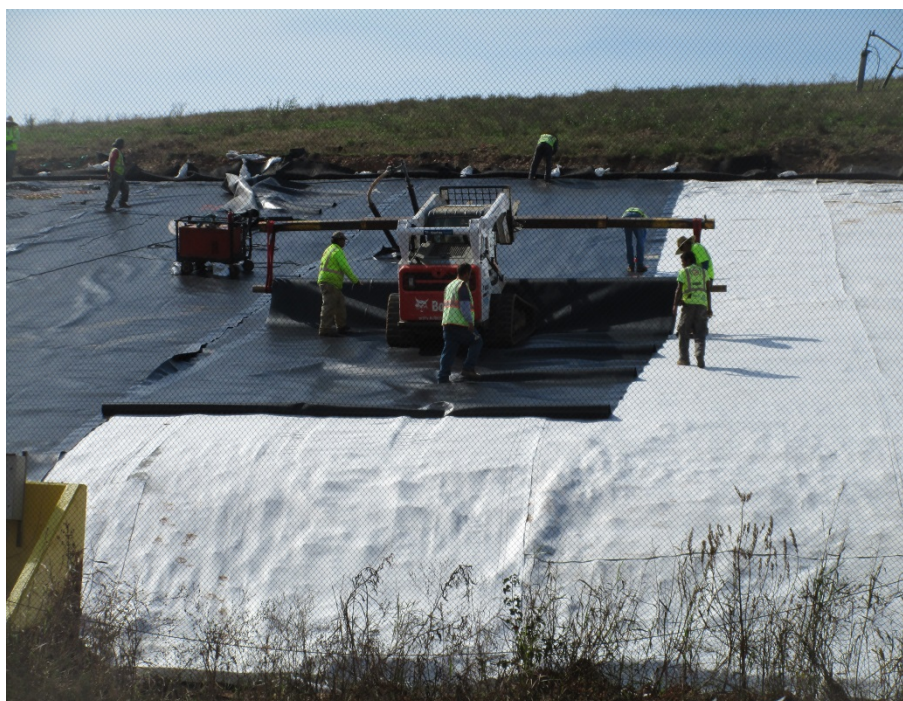
Photo 8 – Deploying 40-mil LLDPE Liner on GCL
