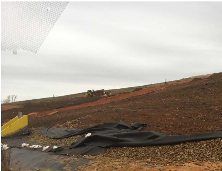
Photo 21 – Hauling, Placing and Grading 12-inch Protective Cover and 6-inch Topsoil Layers
