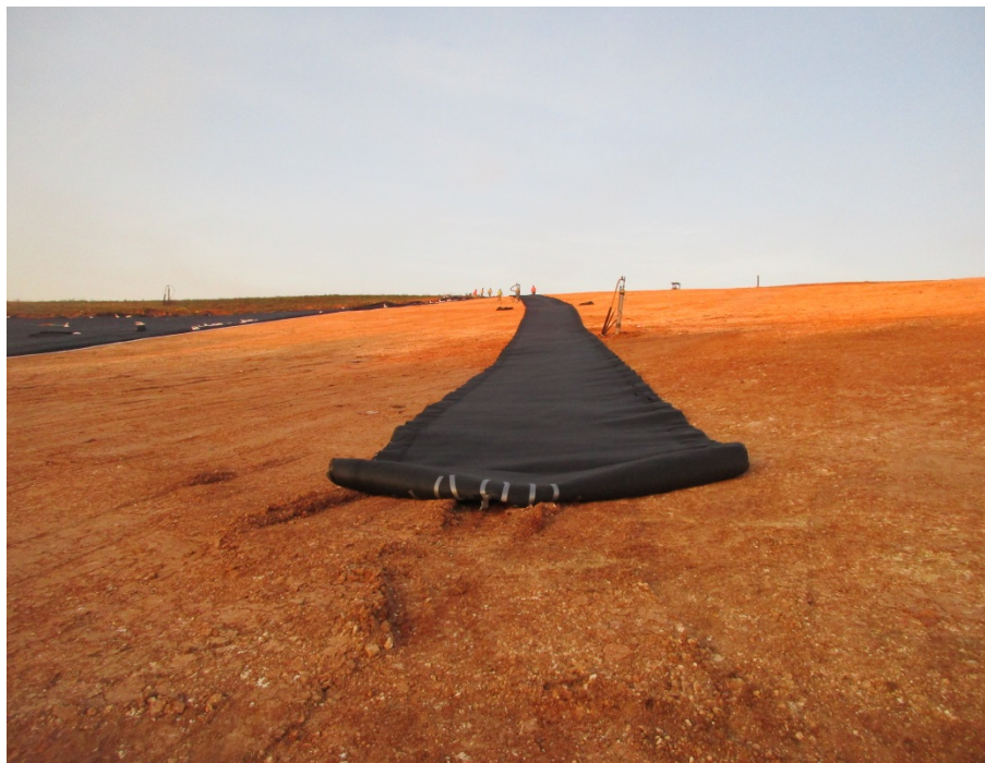
Photo 1 – Installation of the Geocomposite Gas Vent
