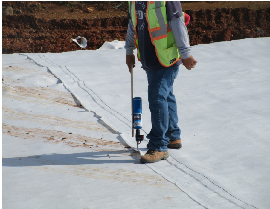
Photo 7 – Heat Tacking GCL Panels Together
