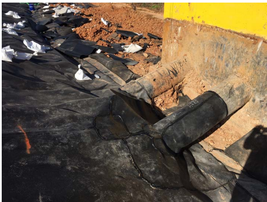
Photo 14 – Extrusion Welded Boots around Cells 1-4 LDS/LCS Riser Pipes at Headwall
