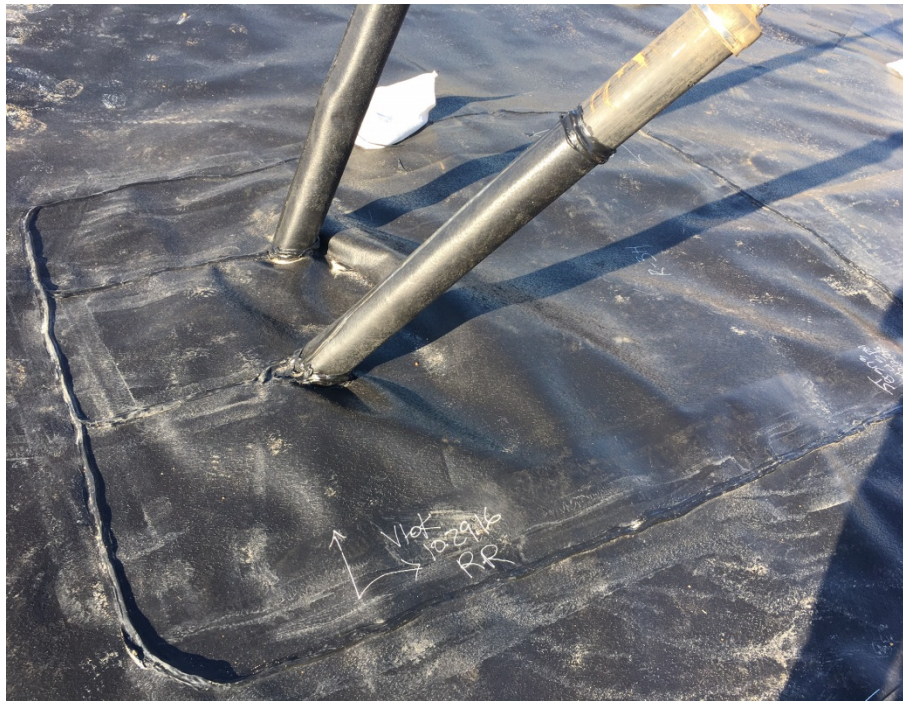
Photo 13 – Finished Patch and Pipe Boots Around Gas Extraction Wells
