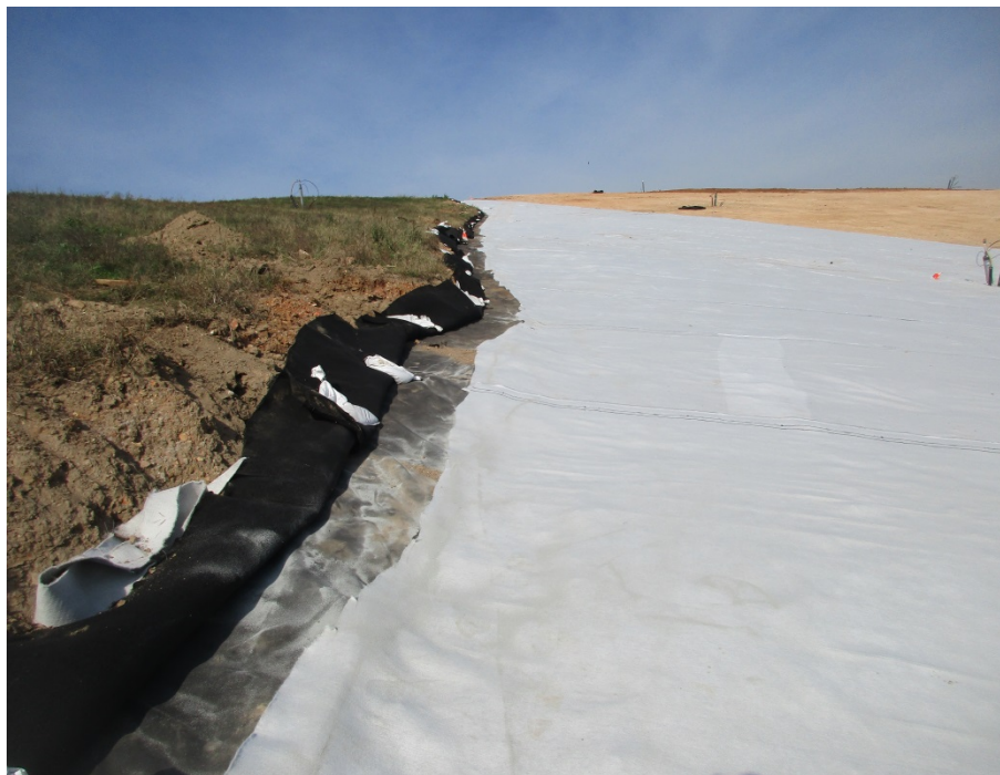
Photo 5 – Placing GCL at South Tie-In to Phase 1
