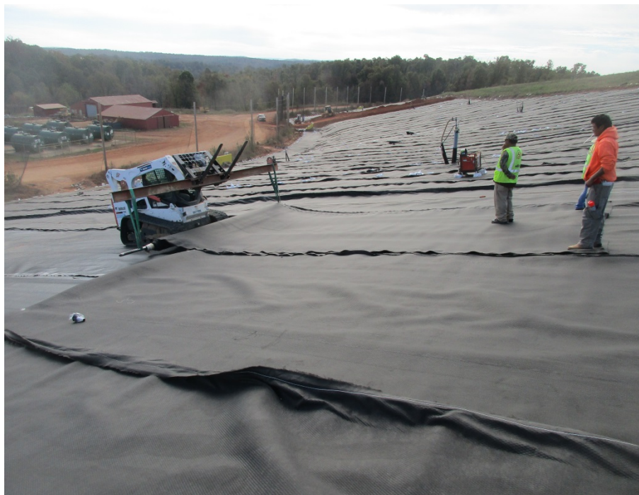
Photo 17 – Placing Double-Sided Drainage Geocomposite
