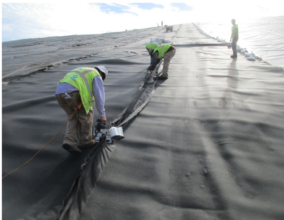
Photo 18 – Sewing Geocomposite panels Together
