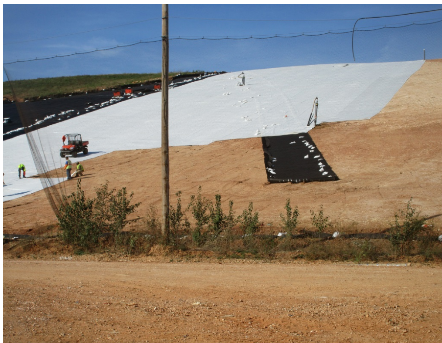
Photo 2 – GCL being placed over the Installed Geocomposite Gas Vent
