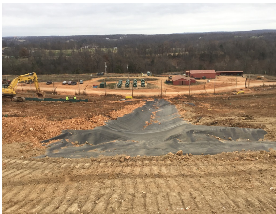
Photo 24 – Letdown on the East Slope Lined with Geomembrane
