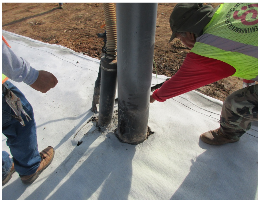
Photo 6 – Heat Tacking GCL in Place at Gas Extraction Wells
