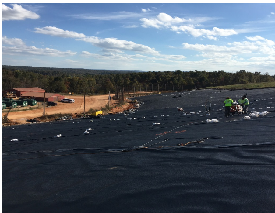
Photo 10 – 40-mil LLDPE Placed on East Slope of Phase 2 Final Cover
