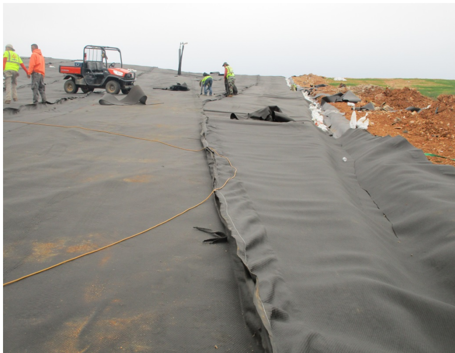
Photo 19 – Completing the Installation of Geocomposite at Termination
