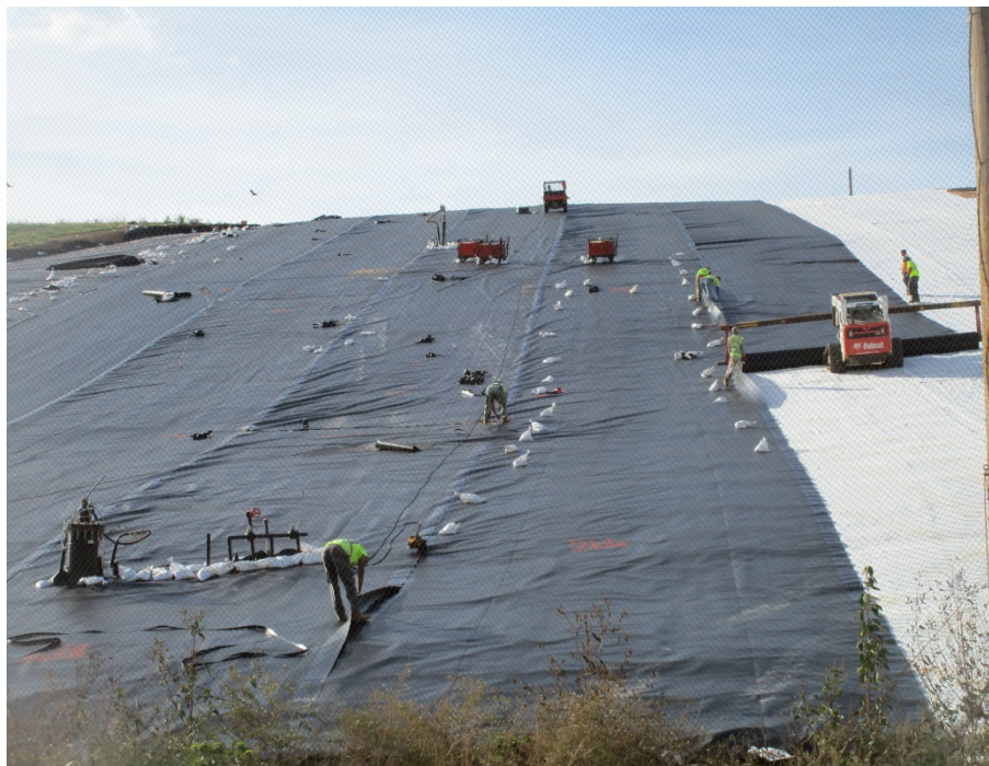
Photo 9 – Deploying and Fusion Welding 40-mil LLDPE on GCL
