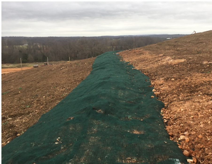
Photo 23 – Completed Drainage Swale with Erosion Control Product
