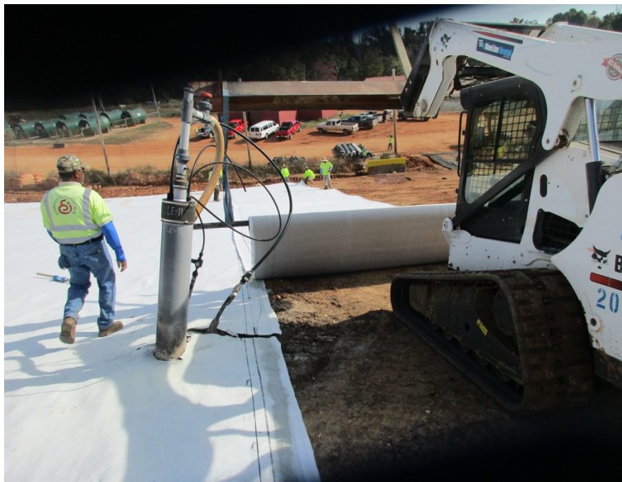
Photo 3 – Deploying GCL on Subgrade
