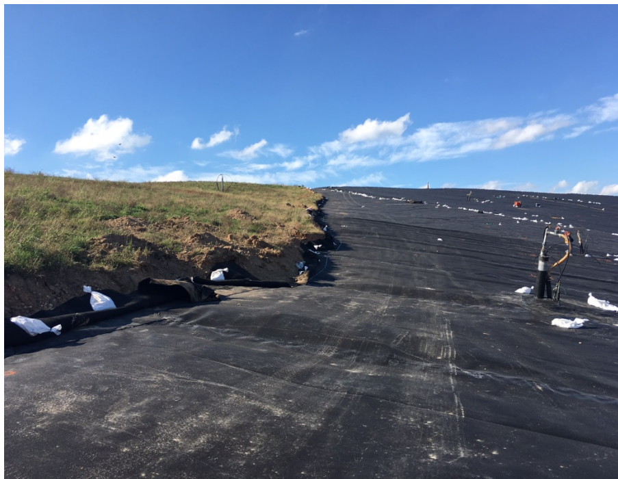
Photo 11 – 40-mil LLDPE Tie-In to Phase 1
