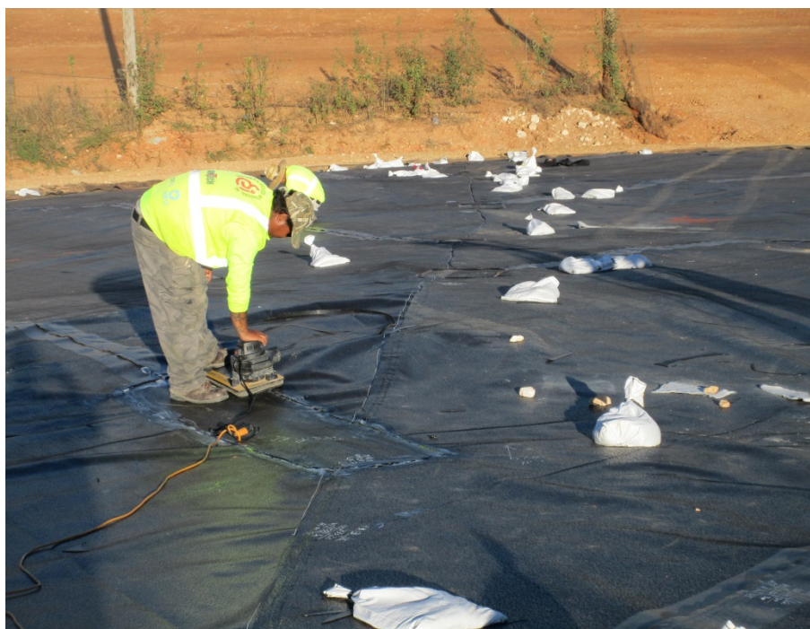
Photo 16 – Vacuum Testing Repairs
