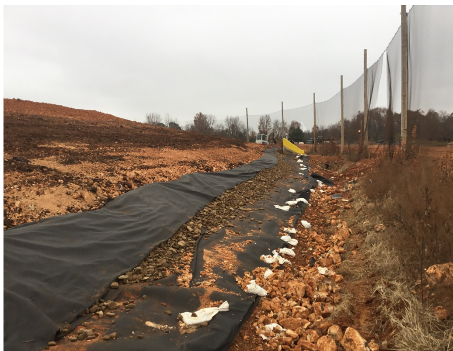
Photo 22 – Finished Installation of Rainflap at Toe of Slope
