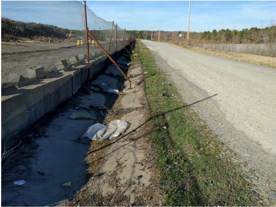
Photo 6: Litter fence and swale
