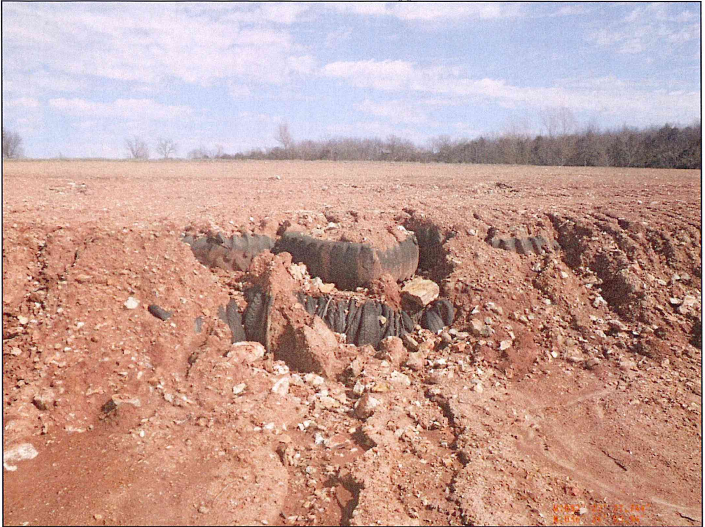
Photo #24: erosion on the upper terrace
