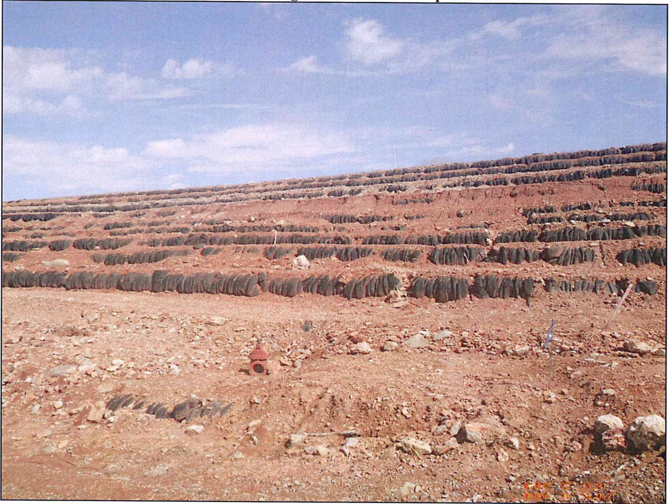
Photo #17: lower terrace right of centerline with pond drain valve
