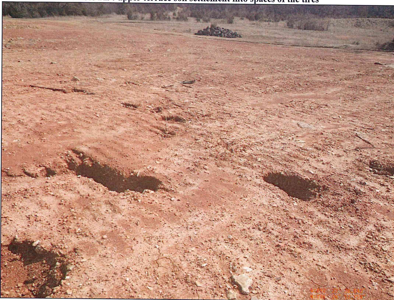
Photo #19: upper terrace soil settlement into spaces of the tires
