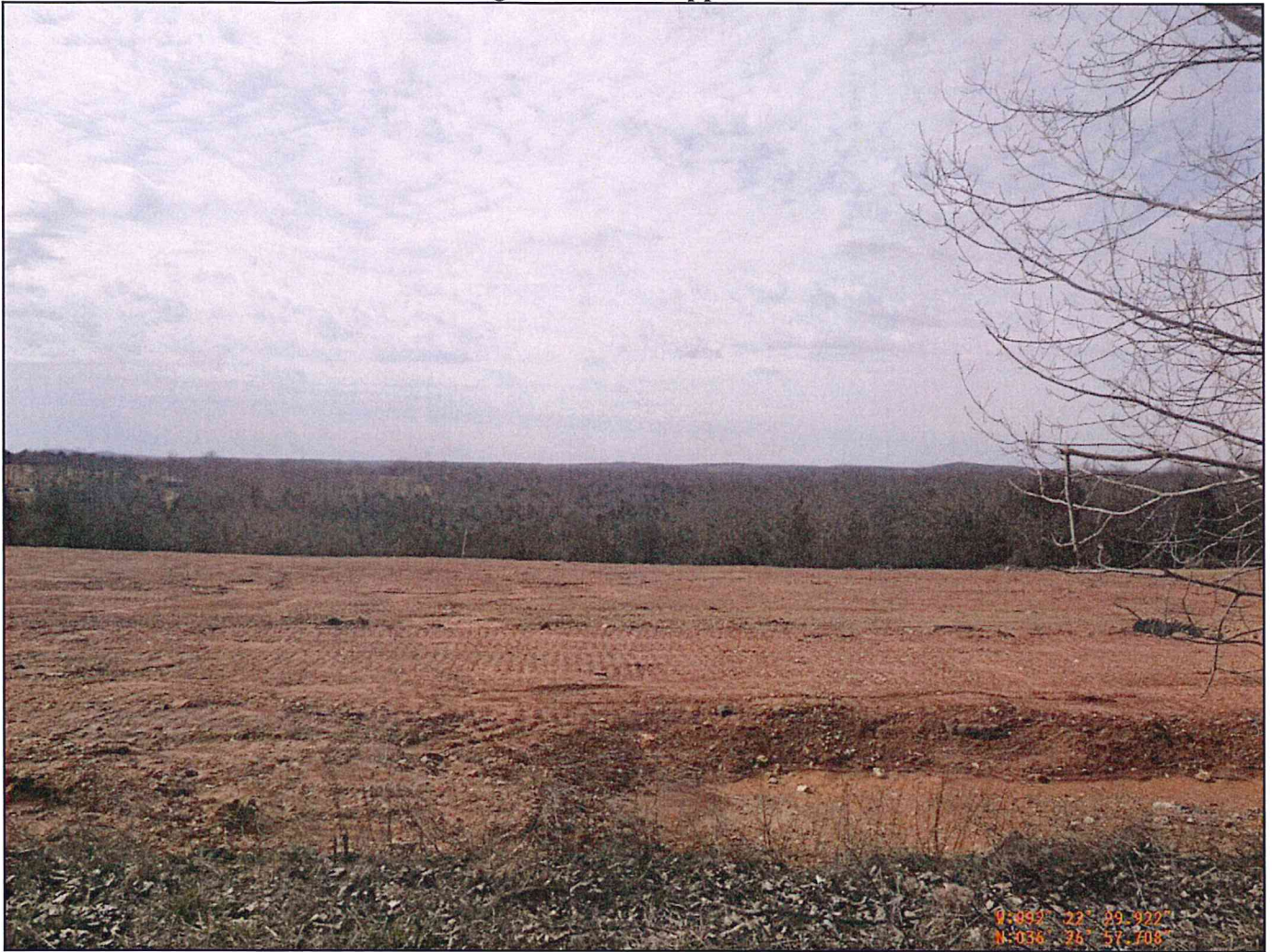
Photo #30: looking down at the upper terrace centerline
