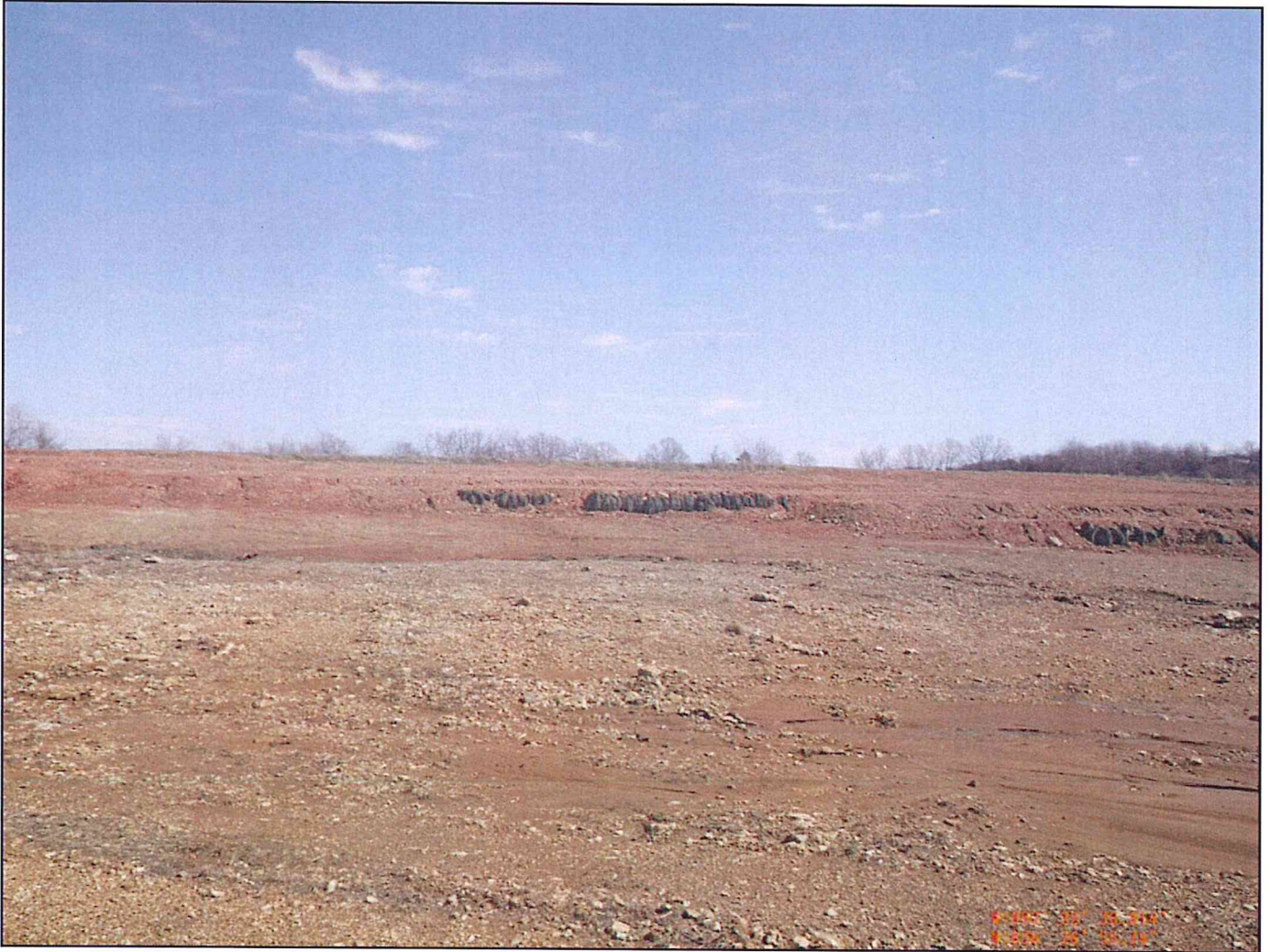
Photo #3: silt fence west road
