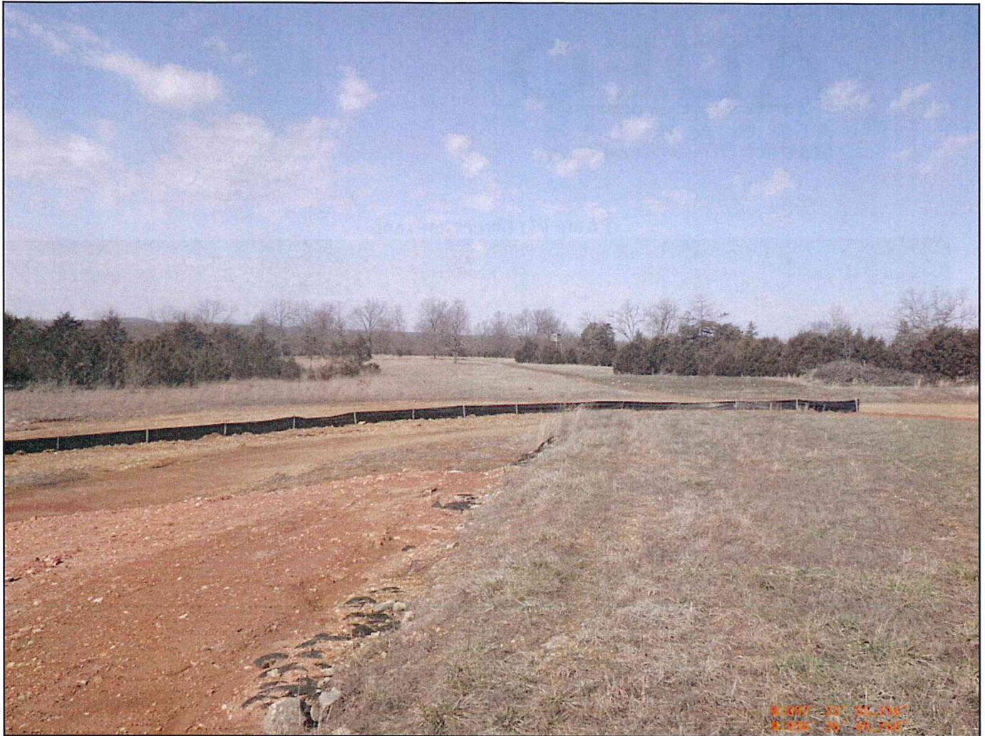
Photo #2: silt fence west road
