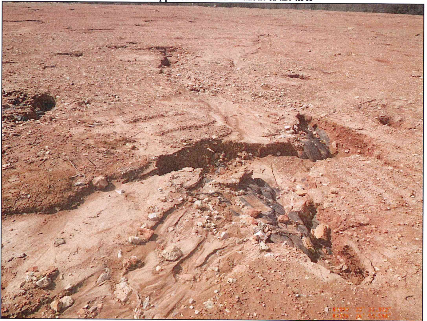
Photo #23: upper terrace soil washout of the tires
