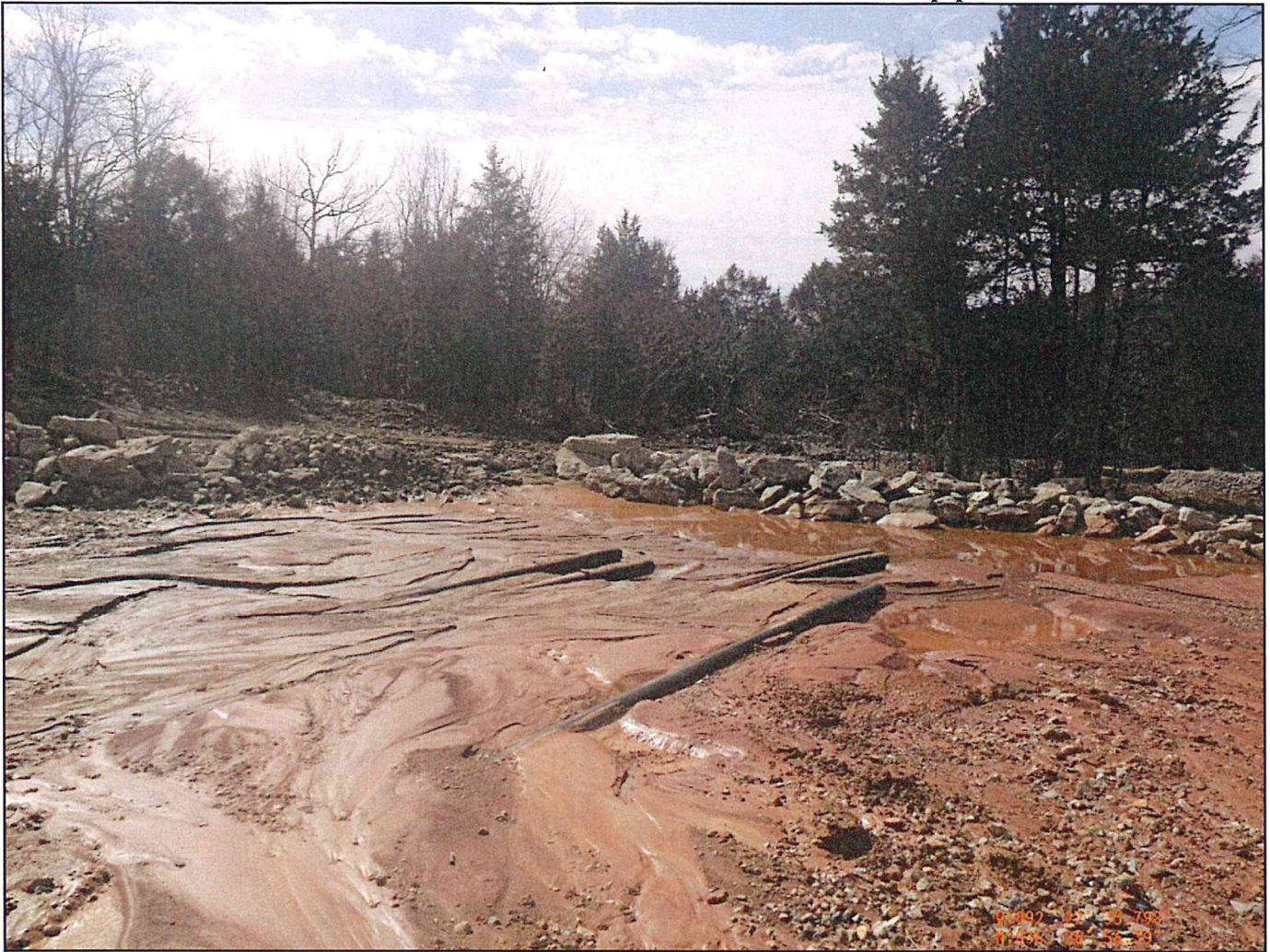
Photo #14: sediment basin toe of the dam at the outlet pipes
