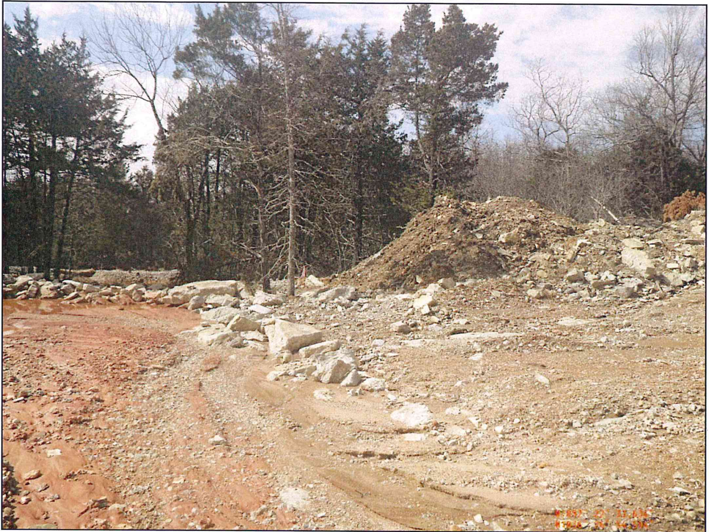
Photo #13: sediment basin toe of the dam
