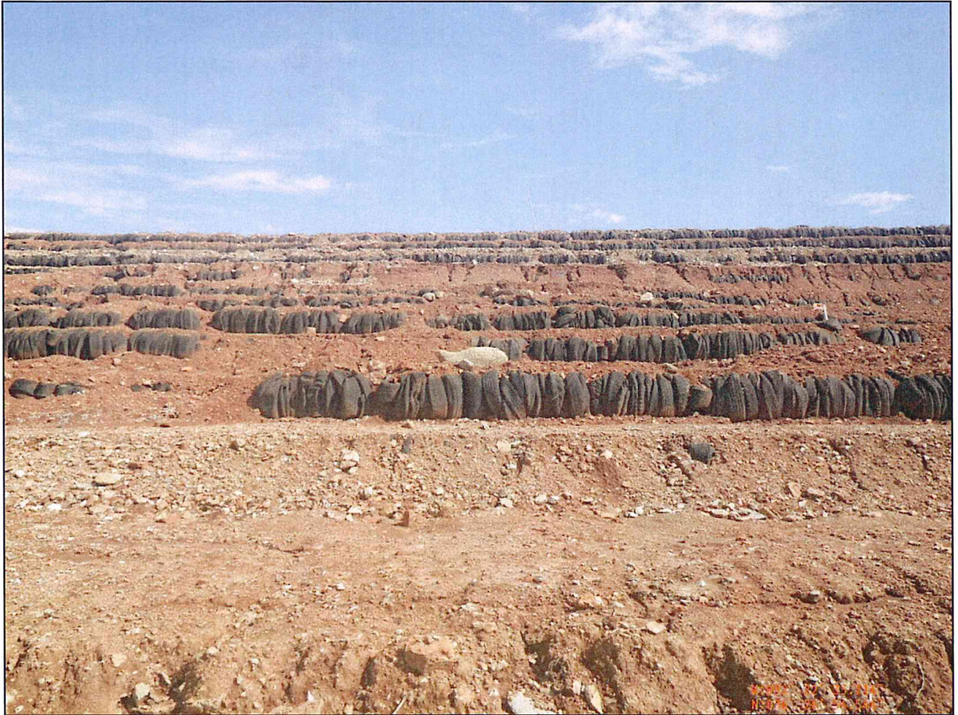
Photo #12: lower terrace centerline
