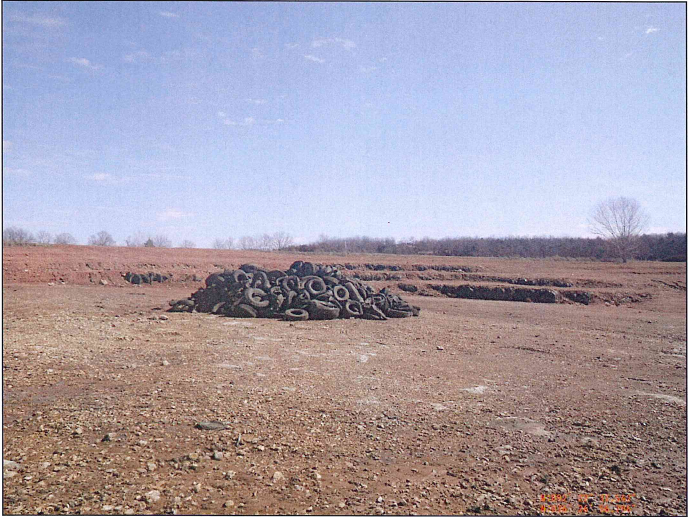
Photo #4: pile of tires on the dam
