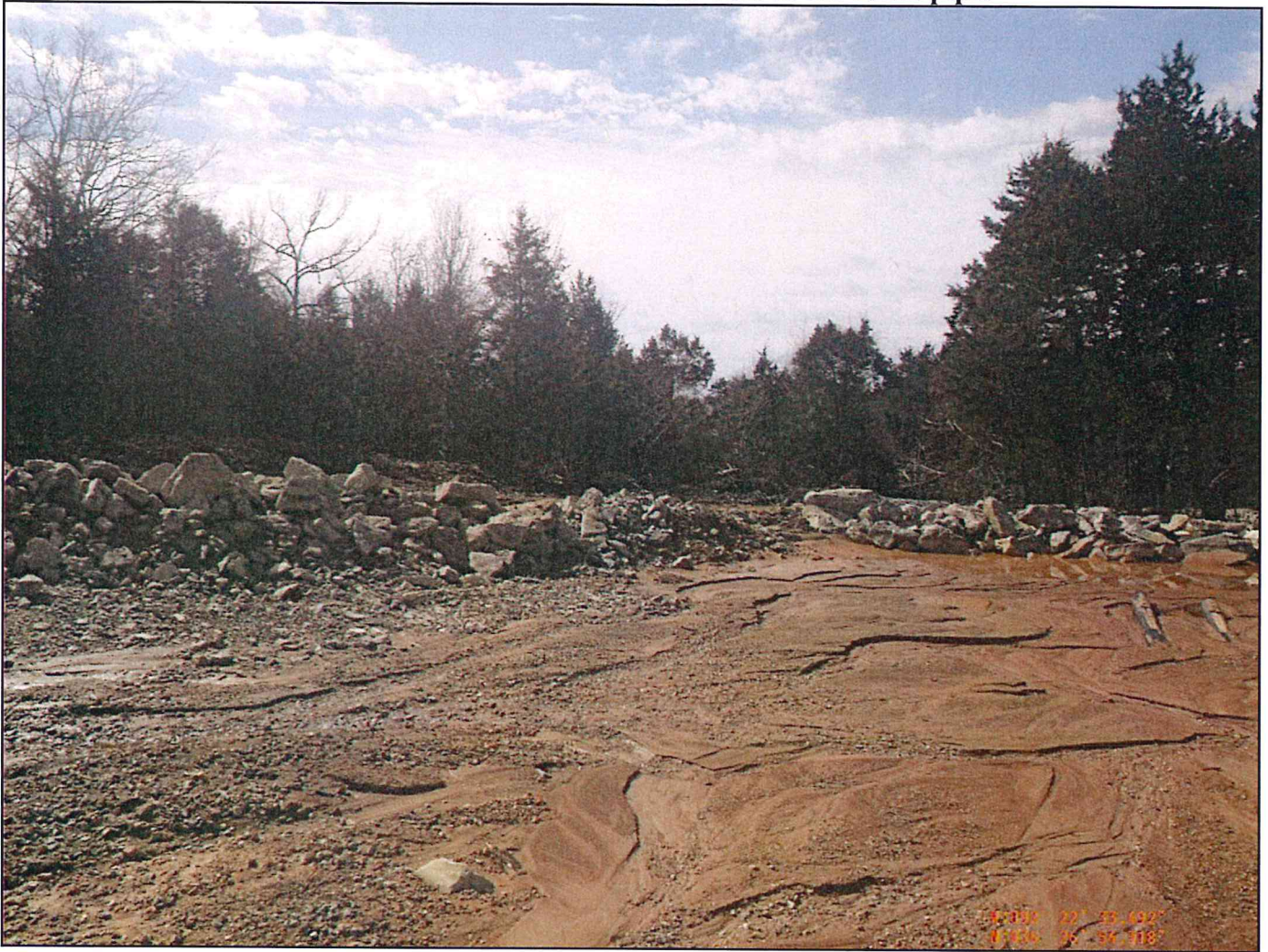
Photo #15: sediment basin toe of the dam at the outlet pipes
