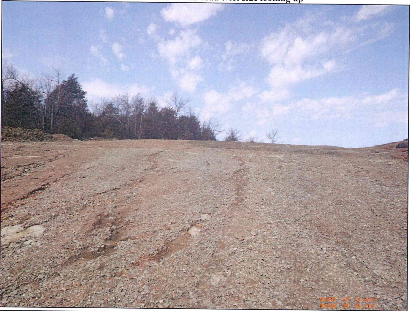
Photo #11: lower access road west side looking up
