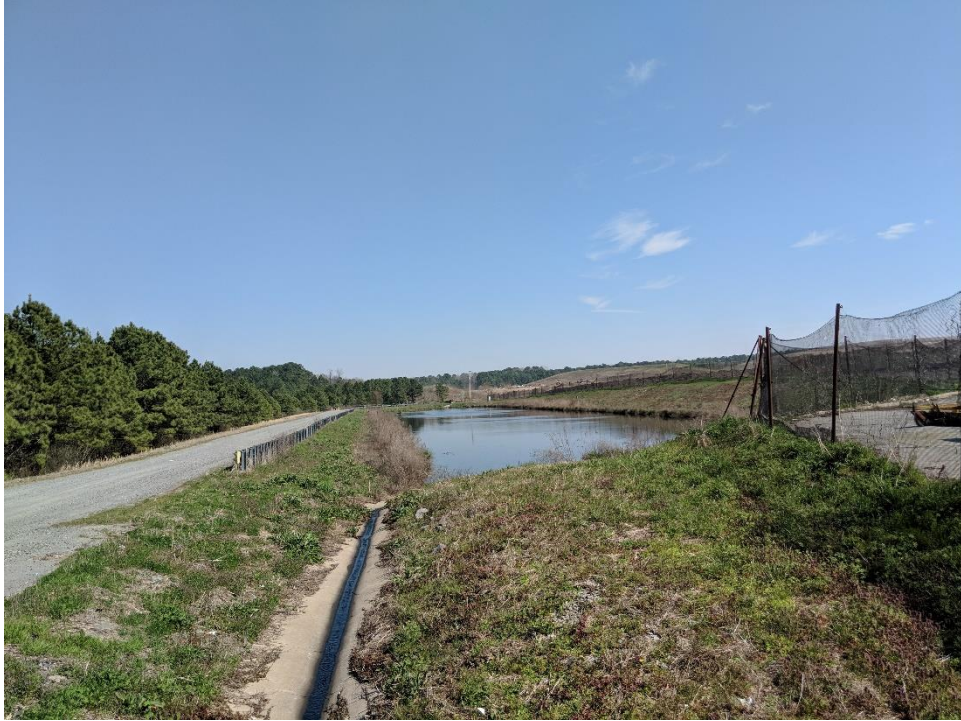
Photo 7: Facility stormwater pond, east side of facility.
