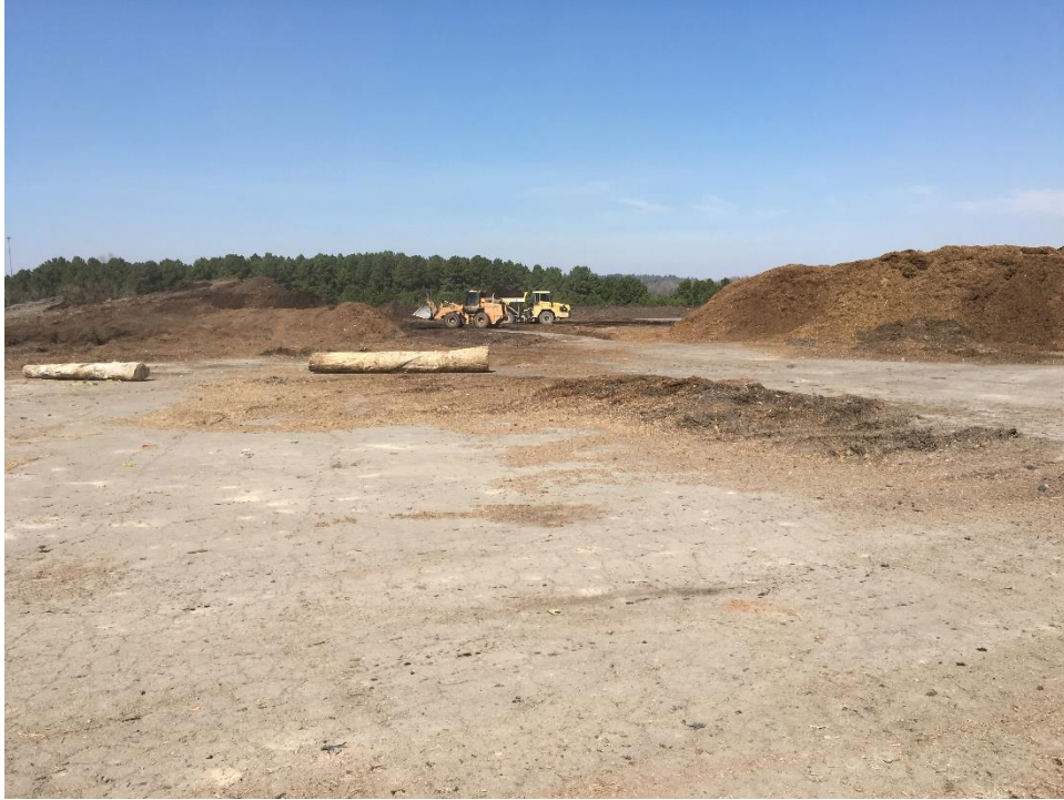
Photo 1: Yard Waste facility from southwest.
