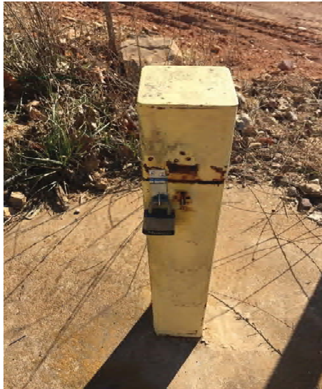
Photograph 4: Groundwater monitoring well MW-1 - new hasp has been added and well locked.
