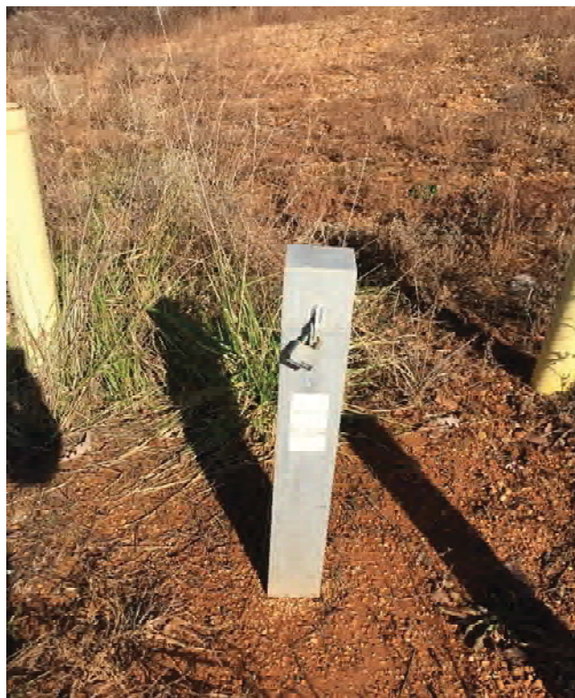
Photograph 9: Groundwater monitoring well MW-5 - locked.
